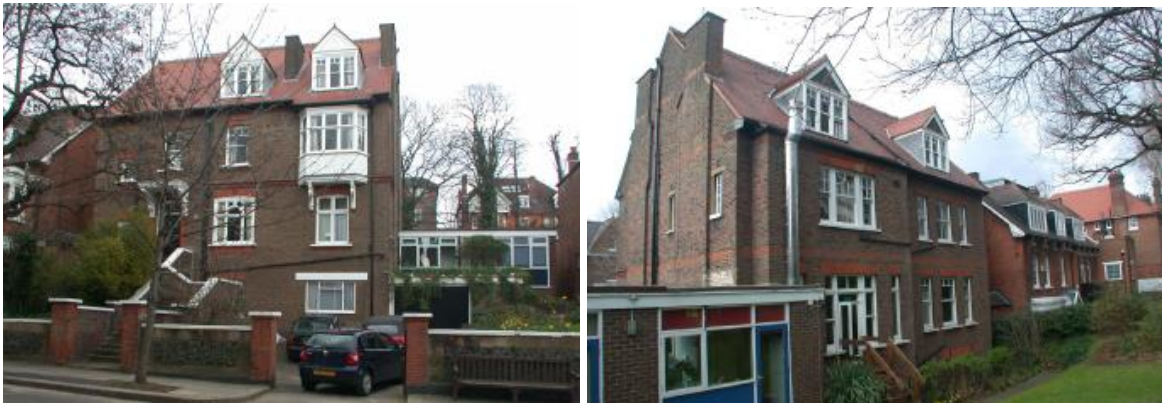
Image – photographs of the existing building showing the 1950s garage structure to be demolished
