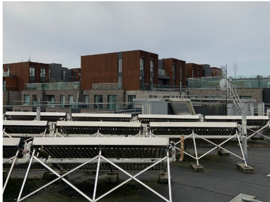
4. View from roof looking across to recently completed Camden Courtyards, 90 St Pancras Way.
