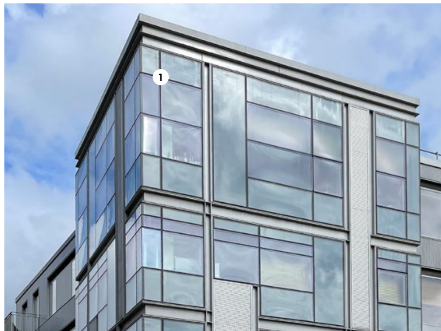
1. Slim framed glazing to the existing "lantern" will be continued in this corner for the fourth and fifth floors.
