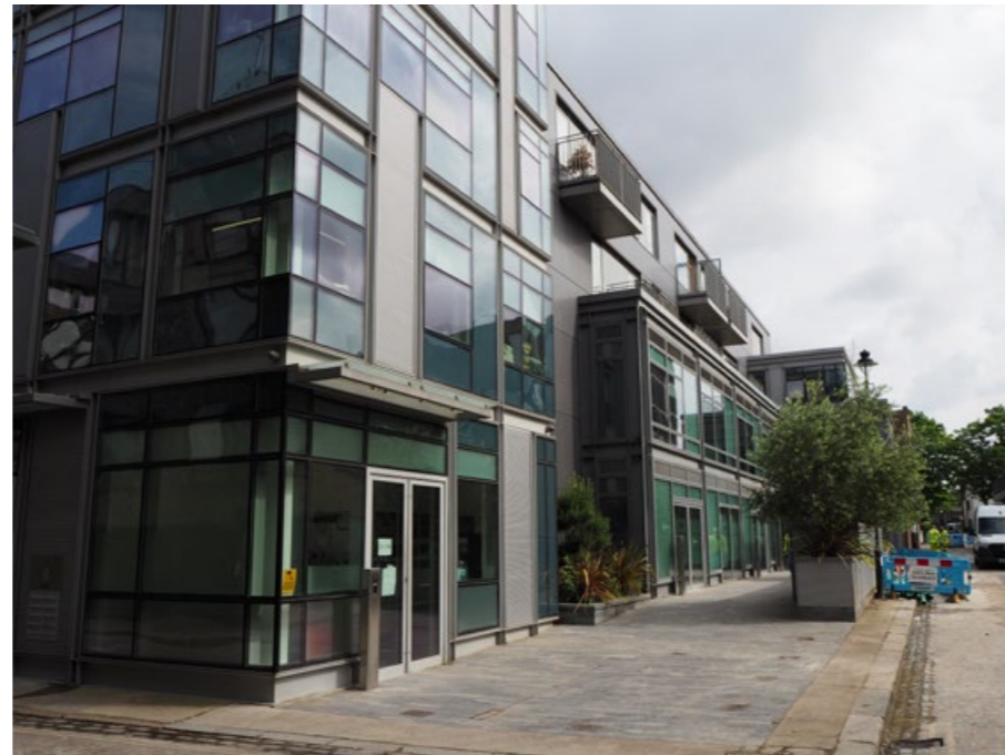
5. View of the existing building looking towards Rochester Road
