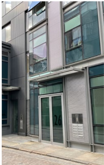
Access from Rochester Place
