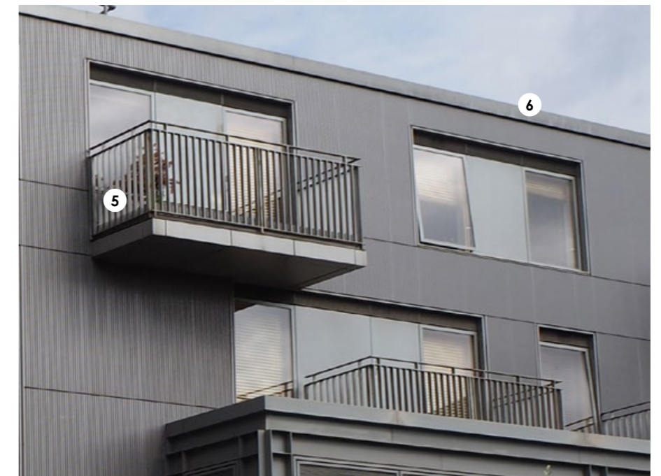
5. Balcony railing on the proposed fourth floor will match the existing floors below 6. Coping to the proposed fourth floor will match those from the existing floors below
