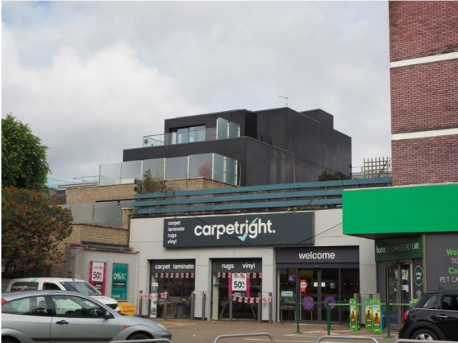
3. Modern four storey residential building backing onto Rochester Mews
