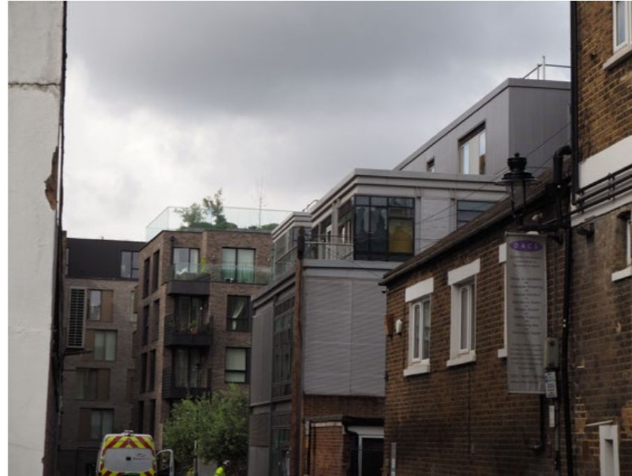
2. View of the existing building along Rochester Mews from Rochester Road
