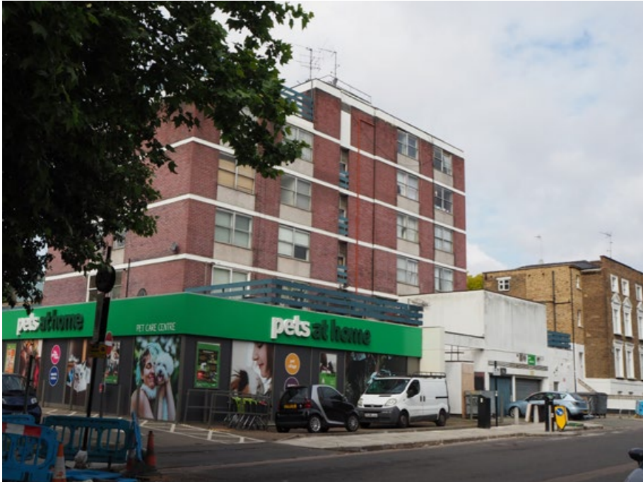
1. Six storey mixed use building on the corner of Camden Rd and Rochester Rd
