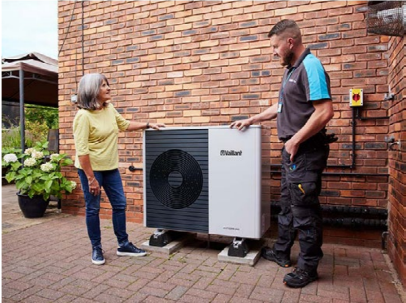
Space has been allocated for potential air source heat pumps www.britishgas.co.uk/
