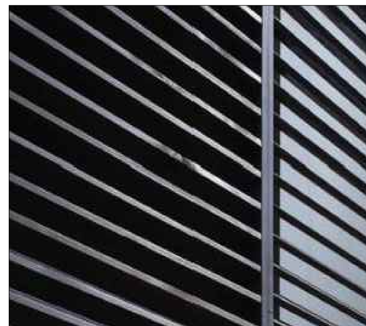
② Ventilation louvre panels above entrance doors
