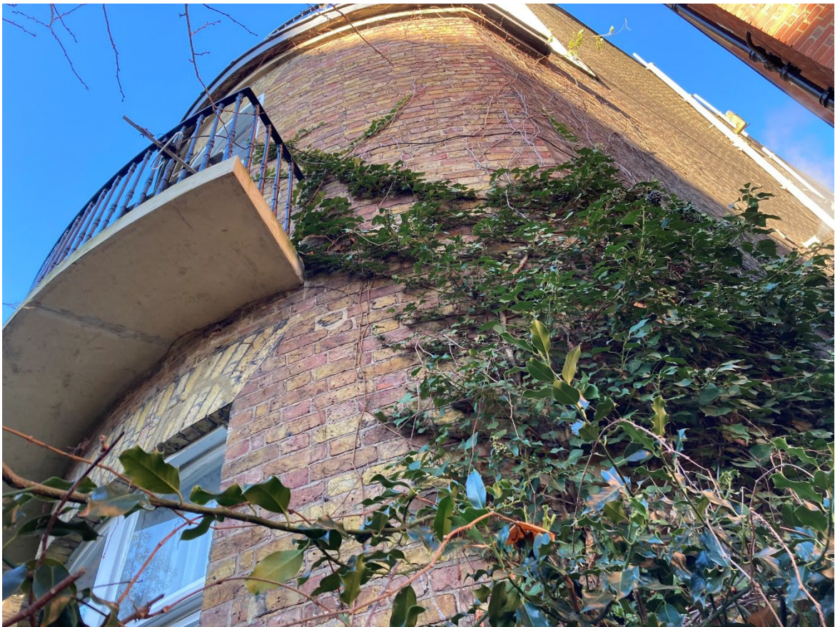
Figure 1 Image of vegetation to the bay window to the rear elevation
