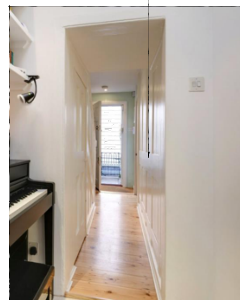
Entrance Hall Photograph Indicating the Removed Panelling to be Replaced on the Right Hand Side of the Photograph
