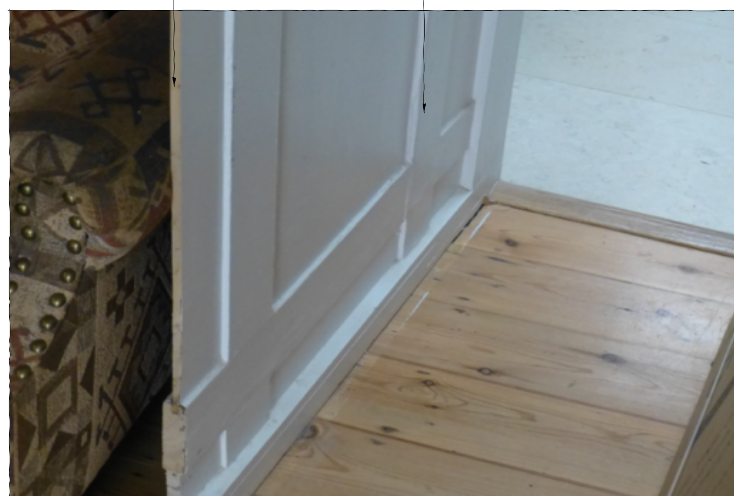
Entrance Hall Photograph Indicating the Section of Retained Existing Wall Panelling
