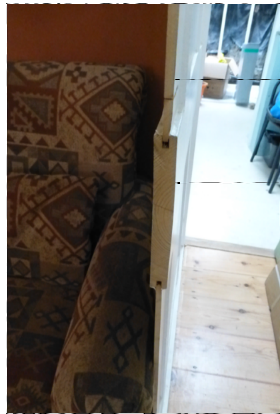
Photograph Indicating Wall Panelling Horizontal Rail with Panels
