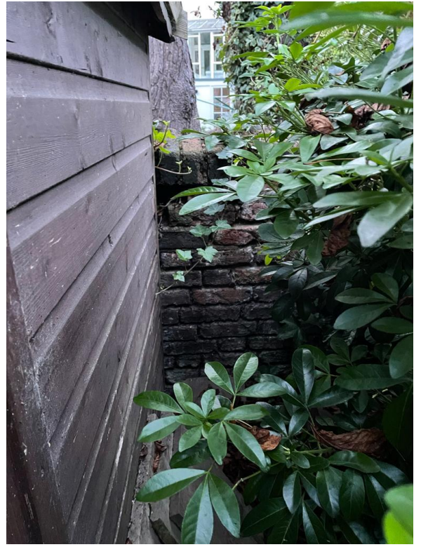
Showing the boundary wall
