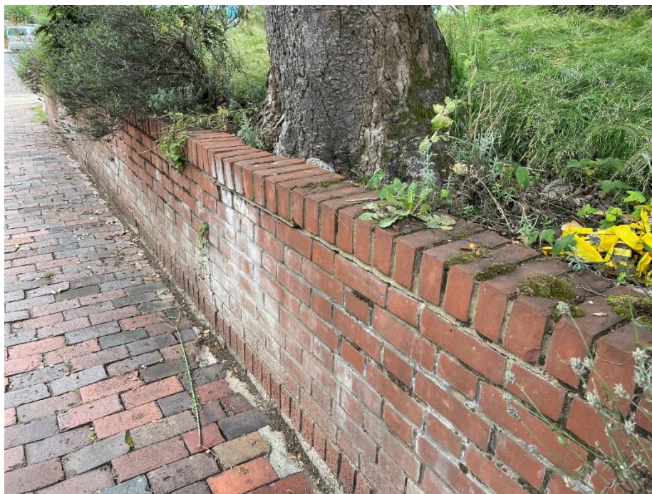
Photo 2 - Leaning wall at tree location
