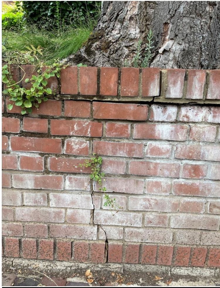
Photo 5 – Cracking at the tree location
