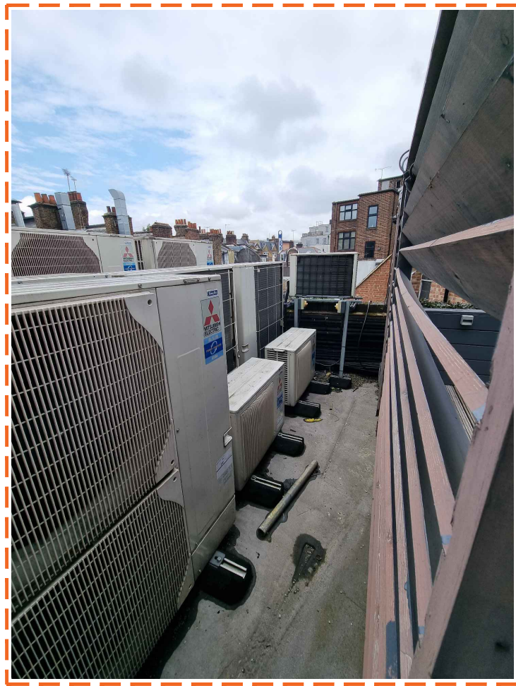
Photo 03 Existing Mechanical Plant retained For use by Gym, Shop & Pub.
