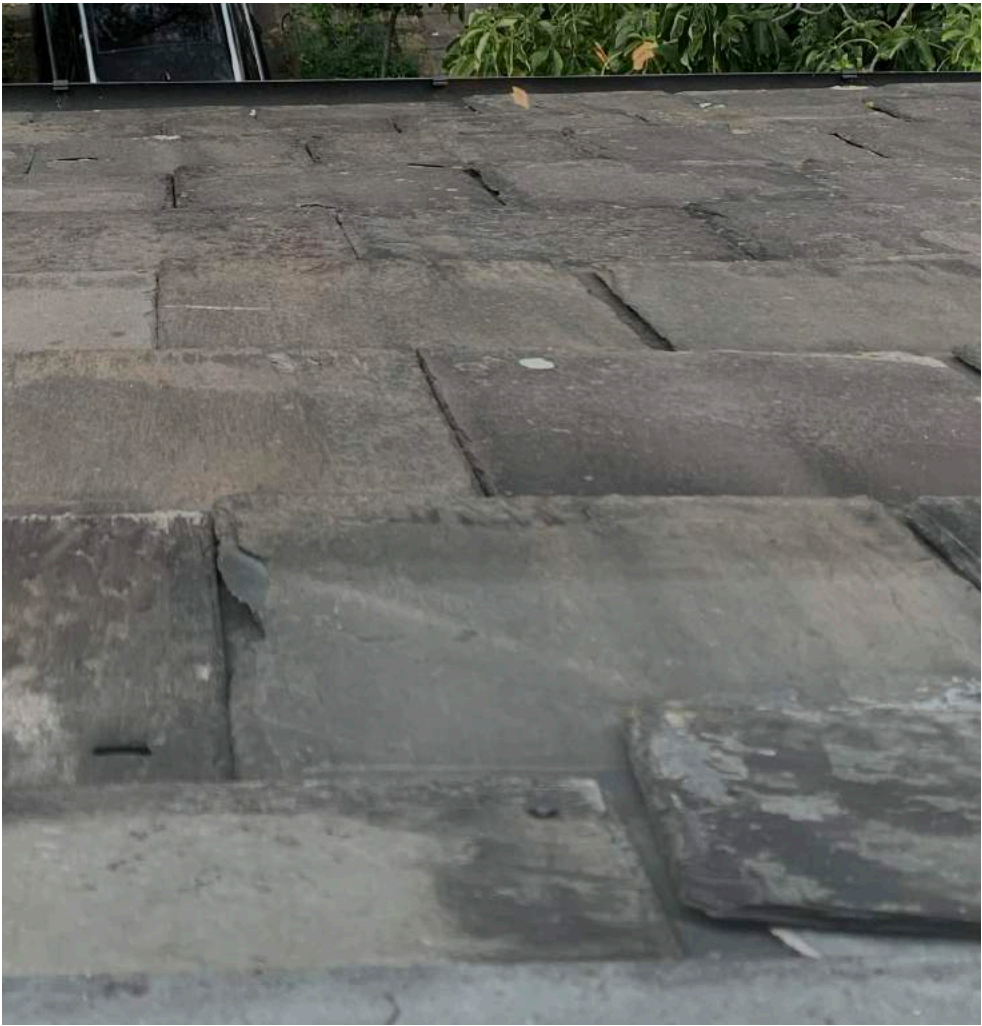
Existing roof. Existing tiles will be removed and brushed/cleaned. Existing tiles to be re-used wherever possible with only broken or defective slates to be replaced.
