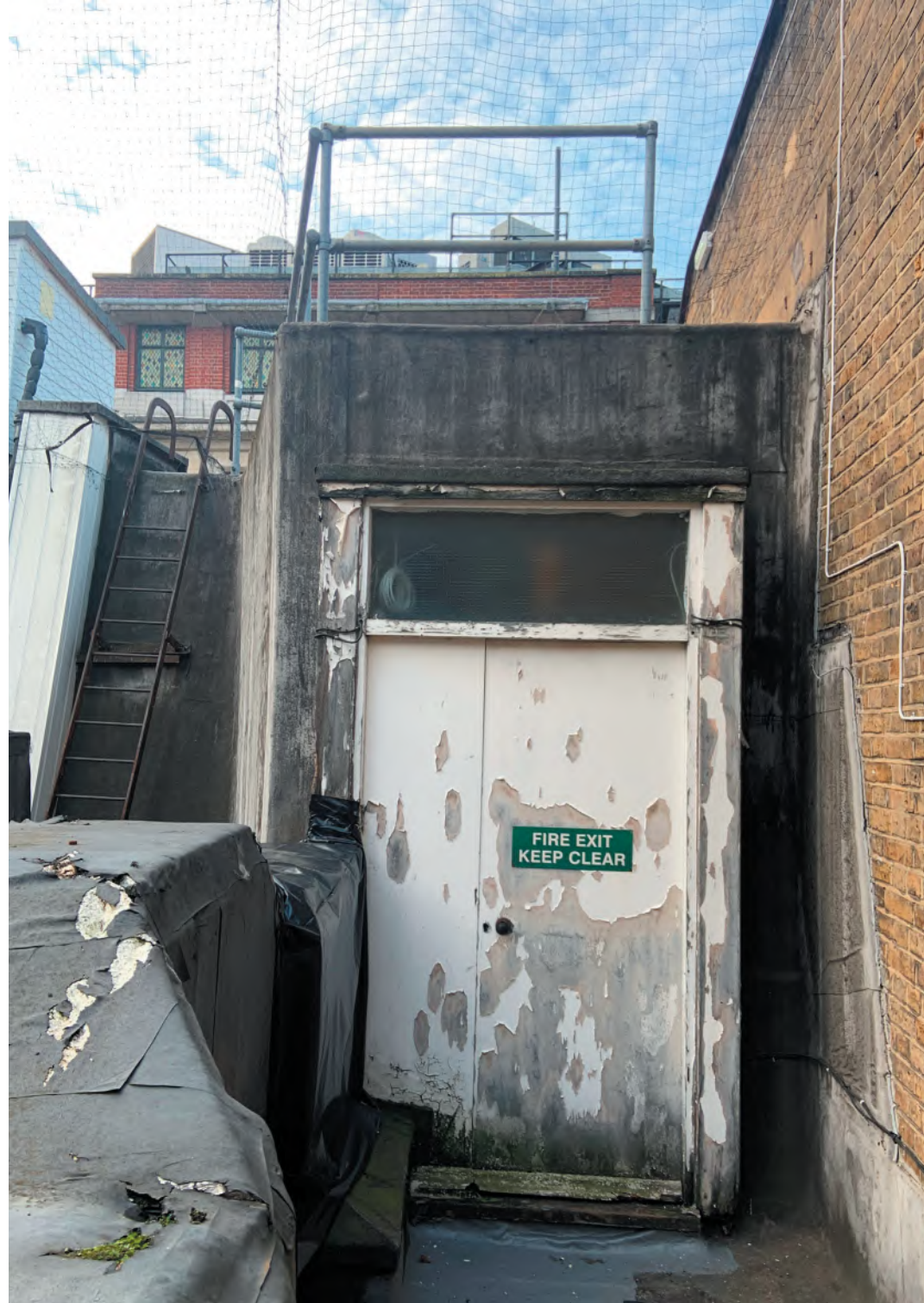
View of the existing dilapidated door from the roof plant outside
