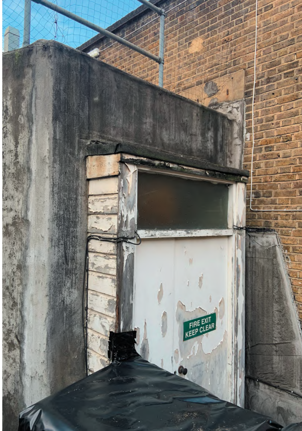
View of the existing door cladding details to be replicated in the new door surrounds
