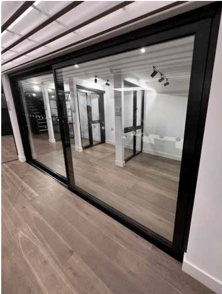
2nd Floor Terrace Sliding Door System: ASE60 lift/slide doors (Schuco Showroom)
