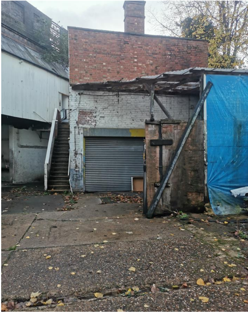
4. View of cottage in rear yard
