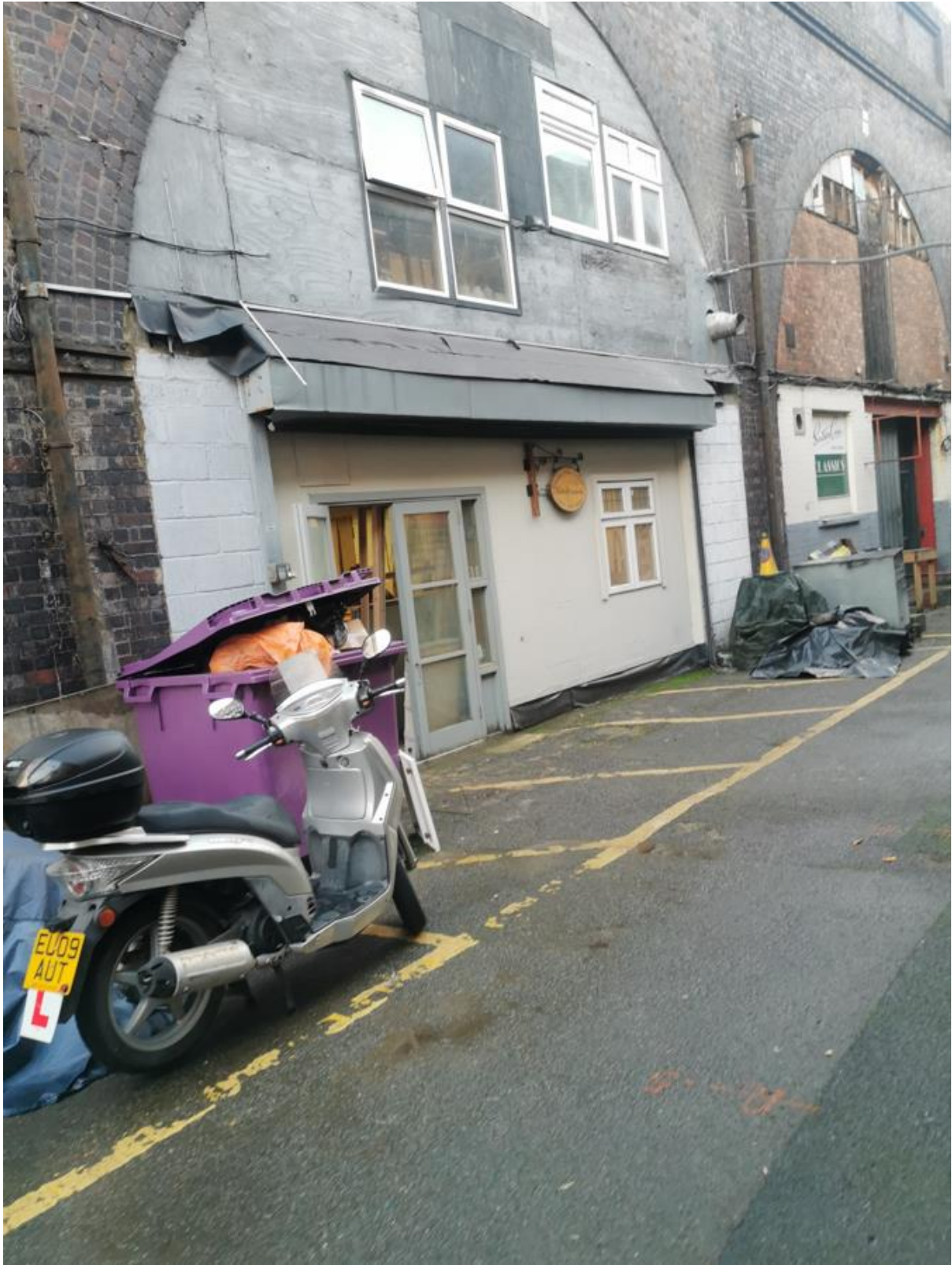
8. Unsympathetic infilling of the arches
