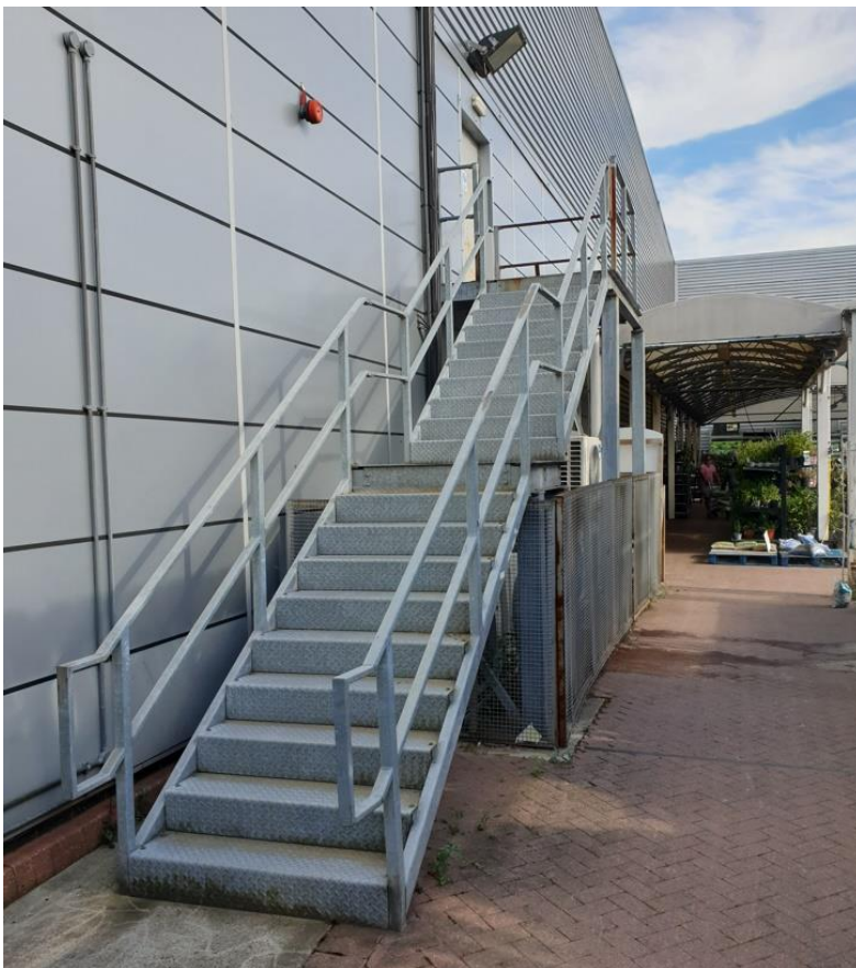
Figure 26 External stairs (fire exit) near the flower garden
