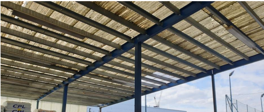
Figure 44 Service yard roofing – GRP panels
