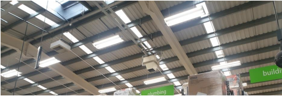
Figure 42 Main building roof – polycarbonate panels
