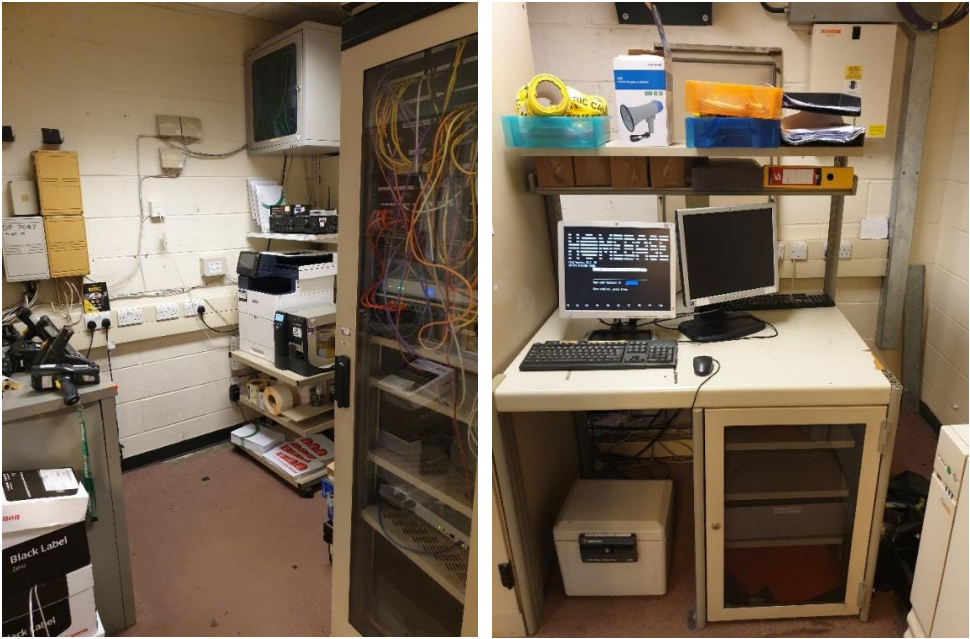
Figure 55 Potential WEEE from the operations room
