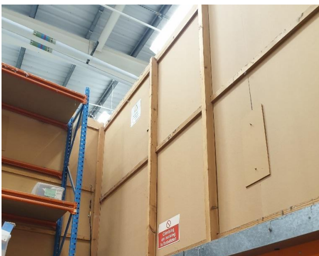
Figure 33 Timber-based panels and framing covering the stock room
