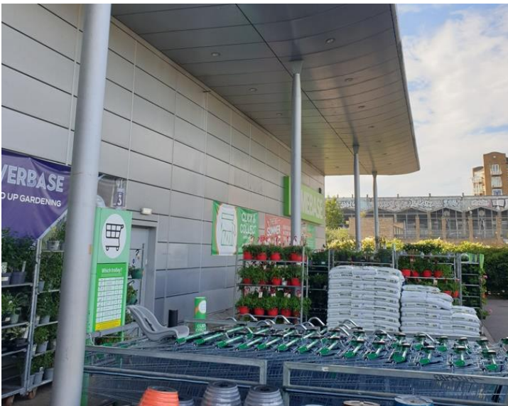
Figure 20 Canopy over main shop entrance
