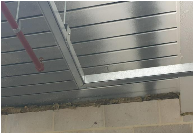
Figure 49 Insulation behind the concrete block wall
