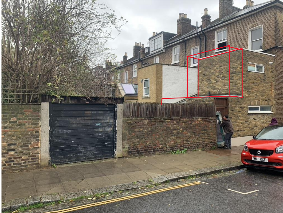
Boscastle Road side elevation: image courtesy of Luke Barclay-Wyand Ground floor, 1.0m extension towards the garden, indicated in red First floor, 1.0m extension towards the garden, indicated in red
