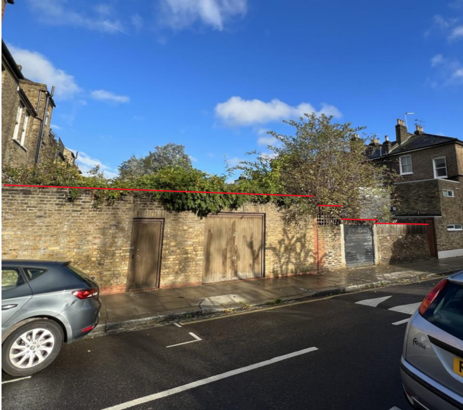
Boscastle Road existing garage elevation: image courtesy of Luke Barclay-Wyand The photograph demonstrates the height of neighbouring brick boundary fence, the height of existing timber trellis adjacent to existing garage and the height of existing garage roof, indicated in red. Also the vertical timber cladding to neighbours existing garage door.
