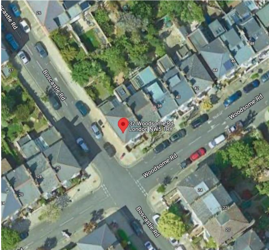
Site Aerial photograph: image courtesy of Google Maps Image shows the original end of terrace house, with 2 story extension to the rear of the house on the Boscastle Road side of the site and a single story glass roof extension adjacent to the neighbouring property at 36 Woodsome Road
