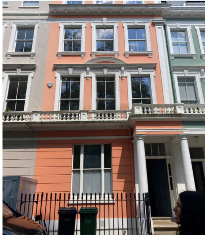
Fig 01 : The front lower portion of 21 Chalcot Square
