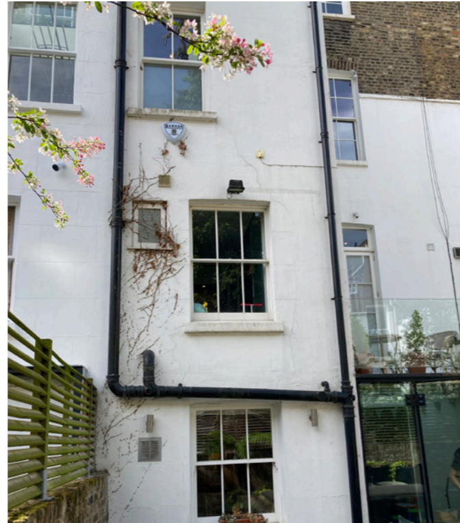
Fig 07 : View of the rear facade - closet wing
