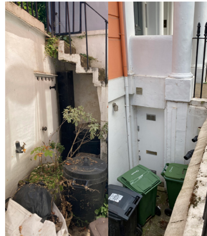
Fig 04 & 05 : Photographs of the front lightwell & steps
