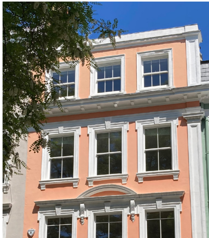
Fig 02 : The front upper portion of 21 Chalcot Square
