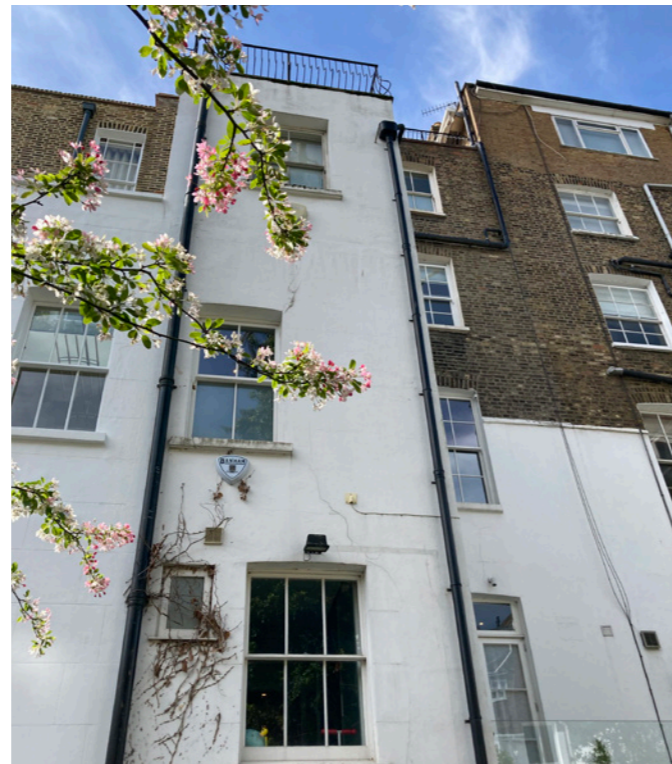
Fig 08 : View of the rear facade - closet wing top
