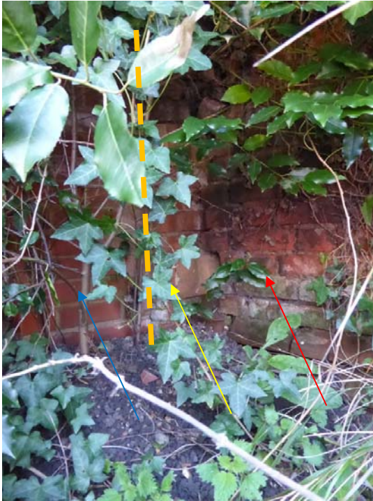
Figure 4 The south boundary wall to The Hoo is indicated in red; the historic brick pier of No. 15/Elim Mansions is indicated in yellow; and the modern brick pier of The Hoo is indicated in blue; and the division between the pier of The Hoo and the pier/ wall of No. 15/Elim Mansions is shown by a dashed orange line
