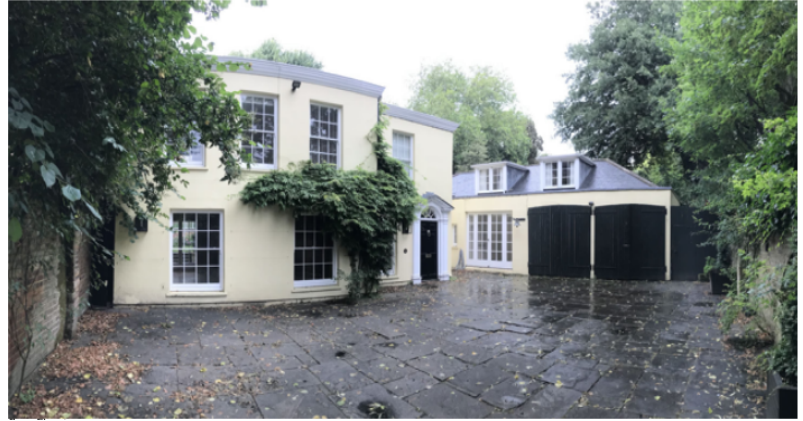
4. Front elevation of existing dwelling
