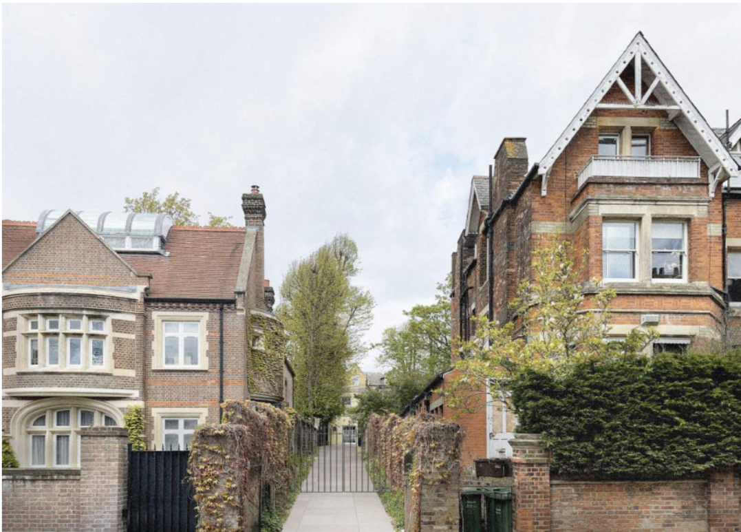
2. View from front to access site
