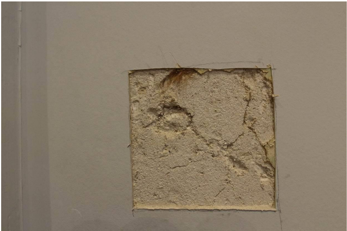
Plate 5 Detail of exploratory opening, showing lime plaster
