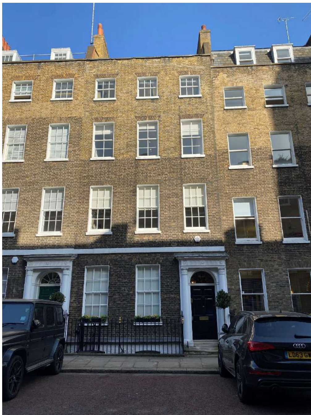
Photo of front elevation of 33 Ely Place
