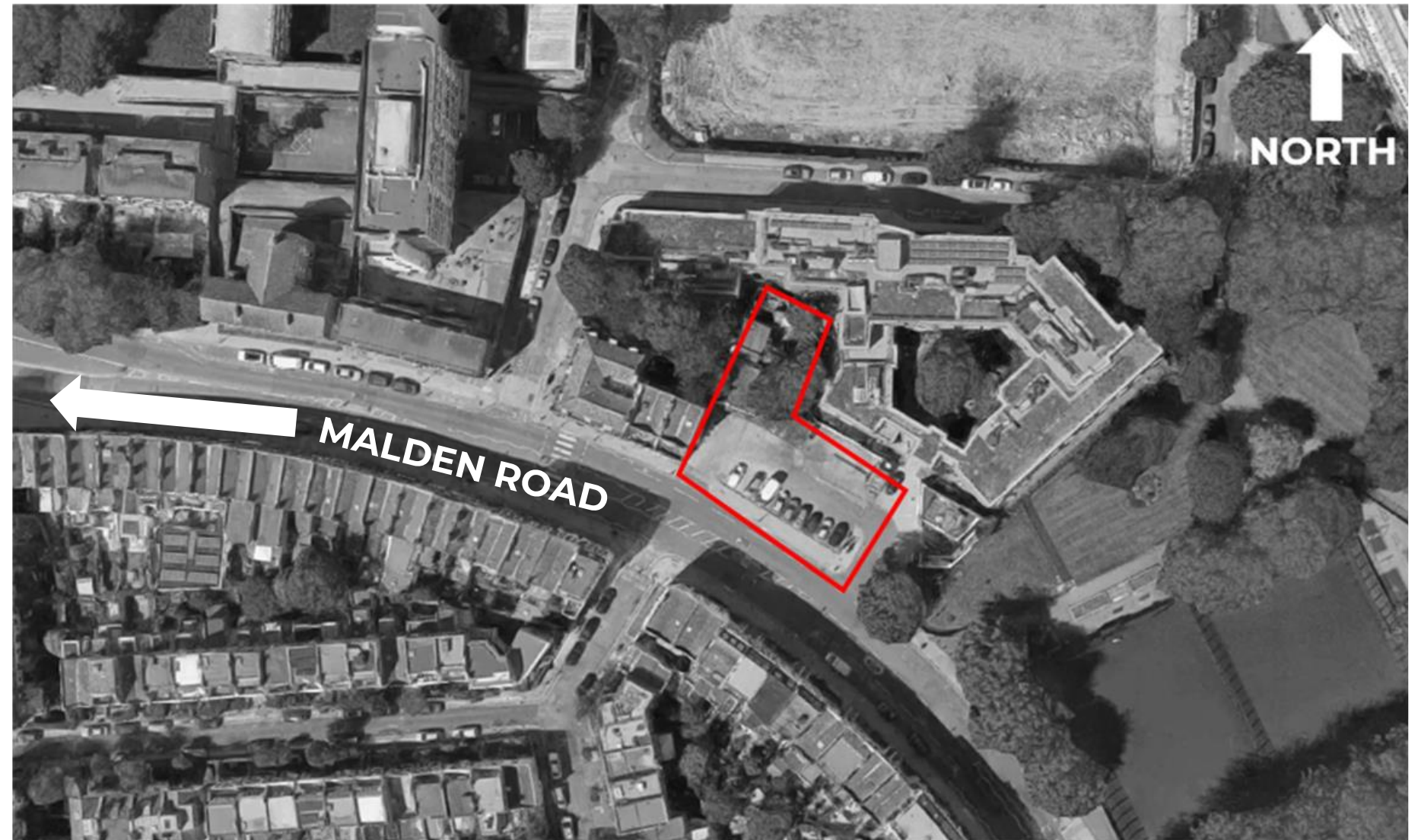
Figure 2: Image of Existing Site (160 Malden Road, Red)
