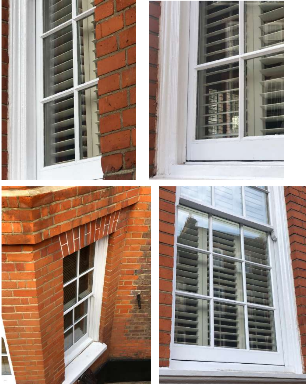
Fig 6.8 – Double-glazed sash windows to the front elevation of Gardnor Mansions
