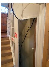
All existing shutters are to be refitted after repairs to windows undertaken. Shutters to be fully redecorated with minor splicing
