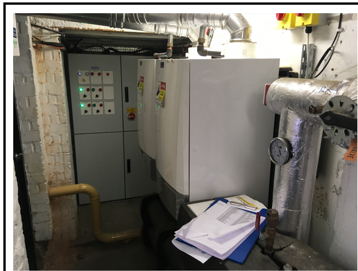
Key internal appliances for removal: Boilers, gas pipework, control panel, pipework. Refer to design access statement for full schedule of works.
