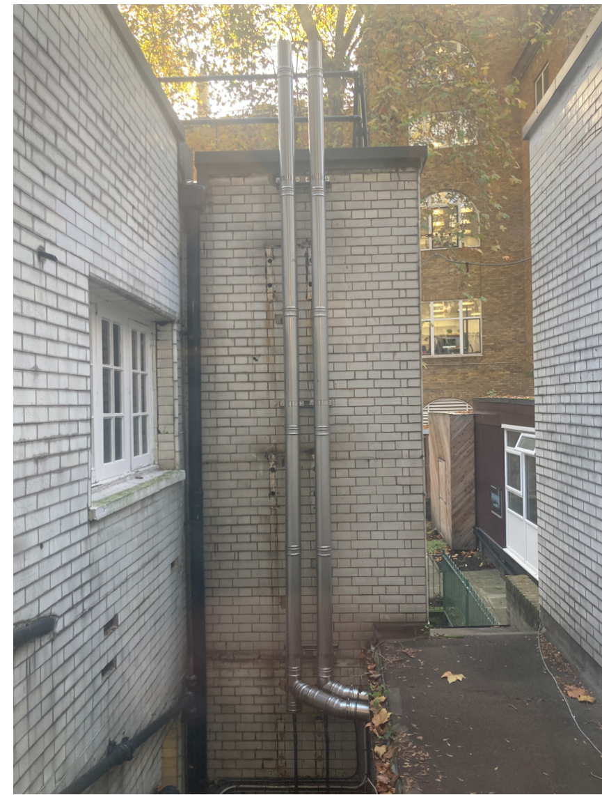
Key external appliances for removal: Gas pipework, flues. Refer to design access statement for full schedule of works.
