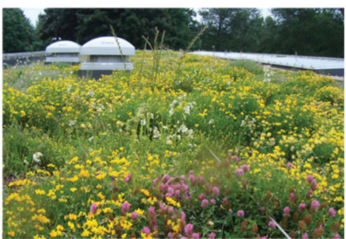
5. GREEN ROOF Intensive Green Roof with deep growing substrate and biodiverse planting of grasses, herbaceous and shrub planting.
