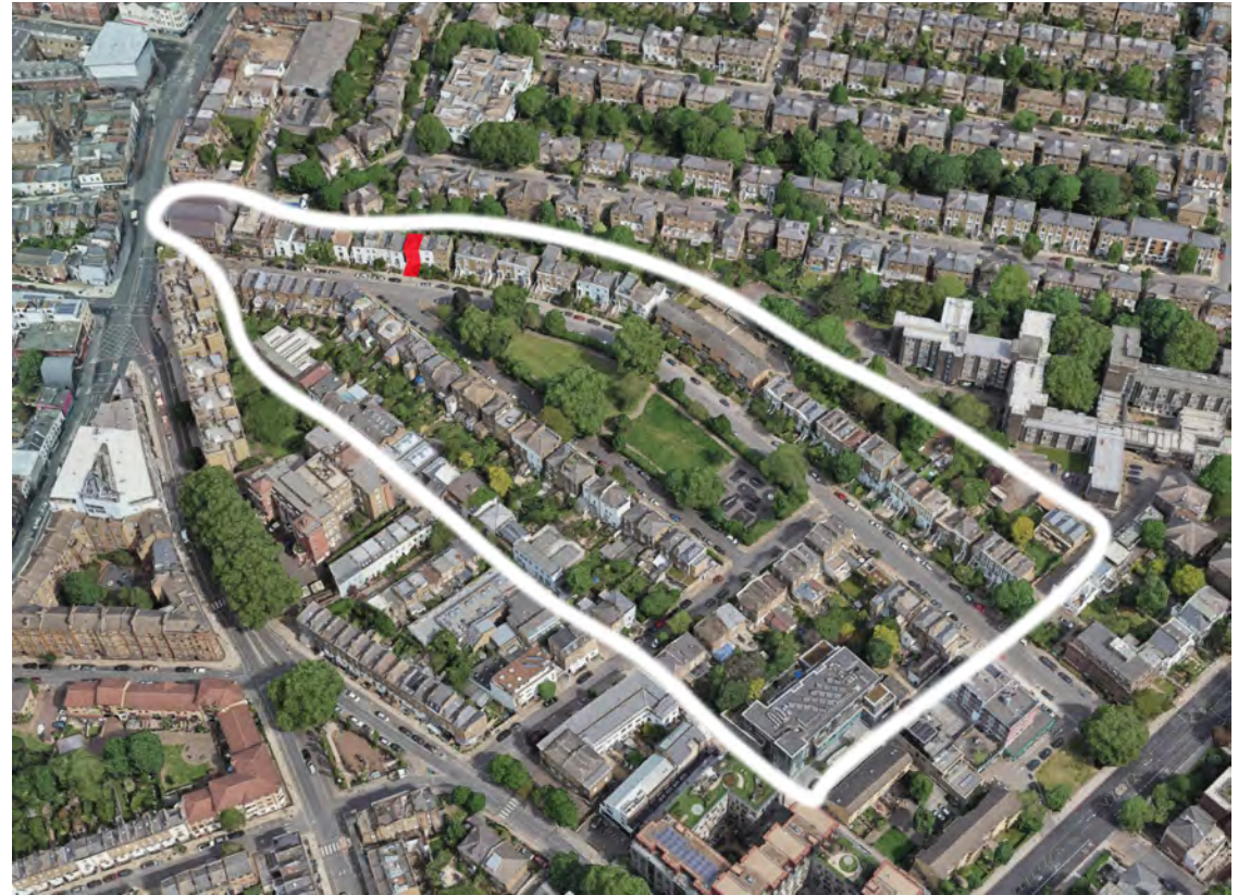
Google Satellite view of Rochester Conservation Area with 35 Rochester Road highlighted in red
