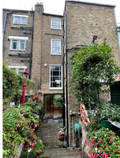
North elevation from garden
