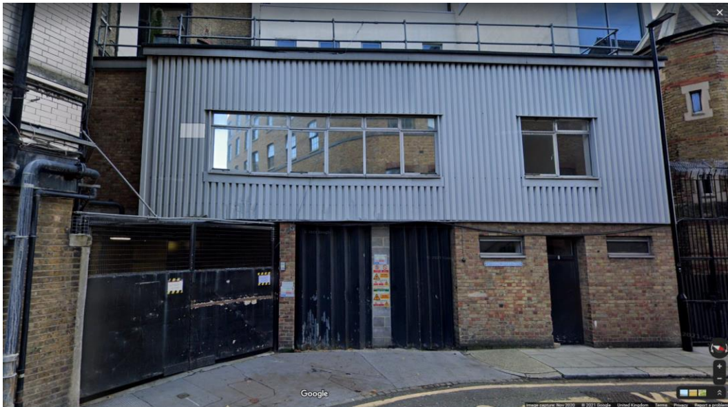
Figure 2: Ear Institute and Service Yard as Seen from Wicklow Street
