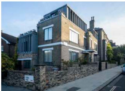
OPTION 3 Option 3 proposes identical brick selection for the main portion of the building. It introduces a slightly darker brick choice at Ground floor level and a Zinc clad top floor.
