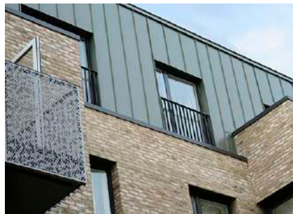
OPTION 3 Option 3 proposes identical brick selection for the main portion of the building. It introduces a slightly darker brick choice at Ground floor level and a Zinc clad top floor.
