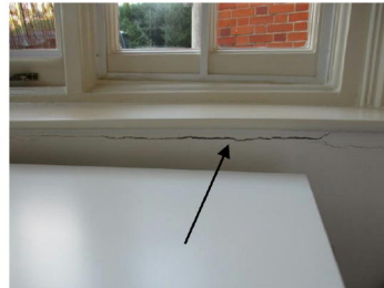
Cracking to bay
