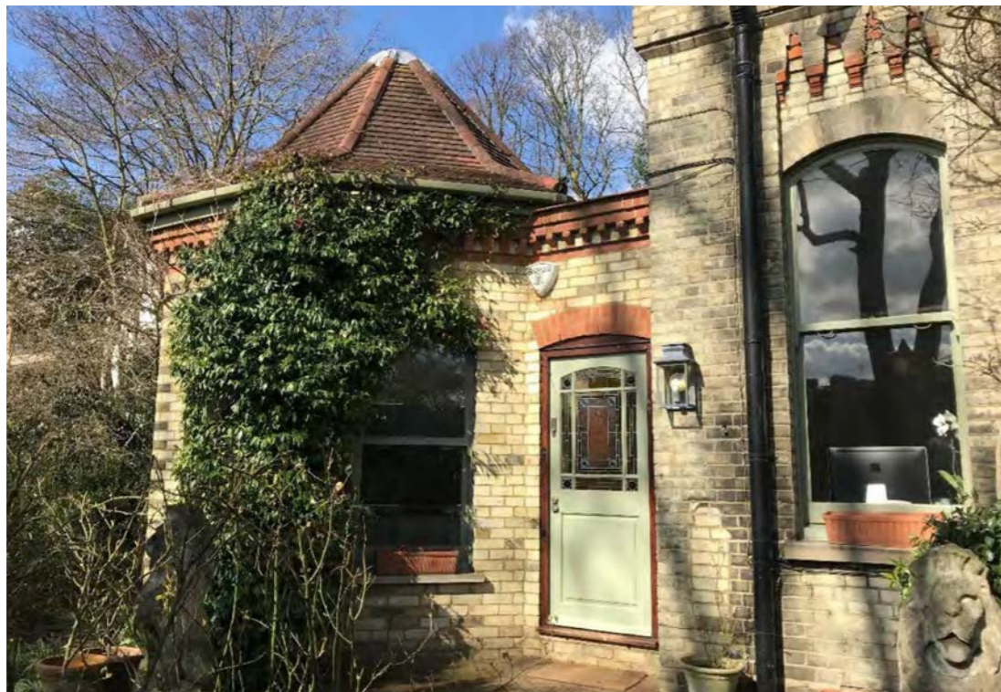
FIGURE 08. Entrance door to 20 Well Road showing both 1950s and 1980s construction
