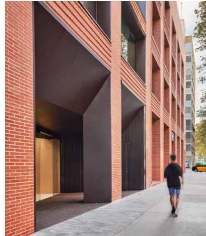
Example metal facade
