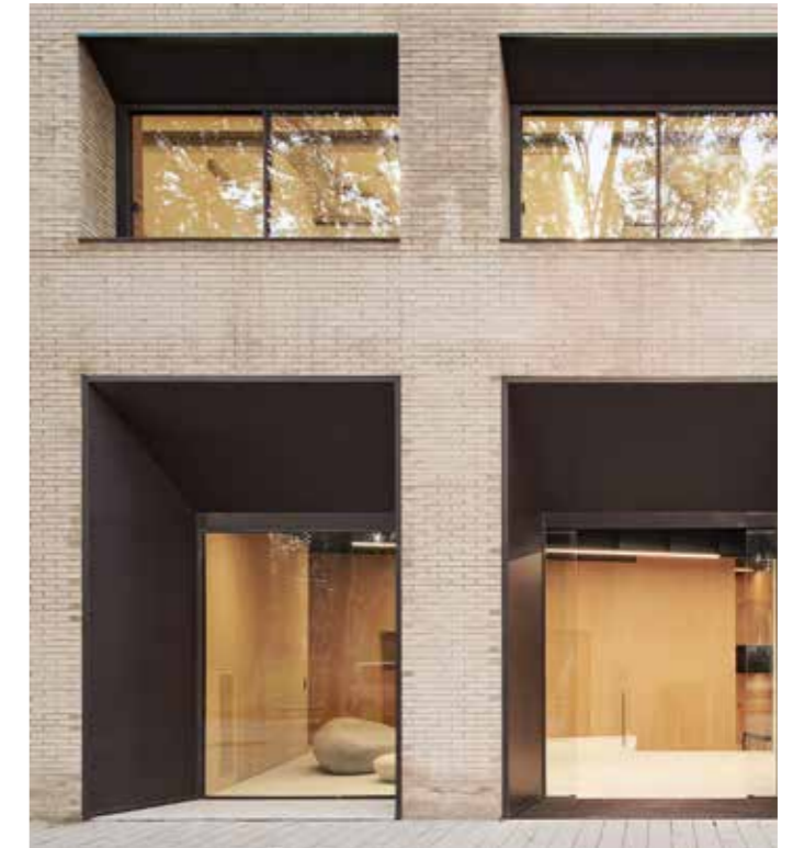
Example metal facade
