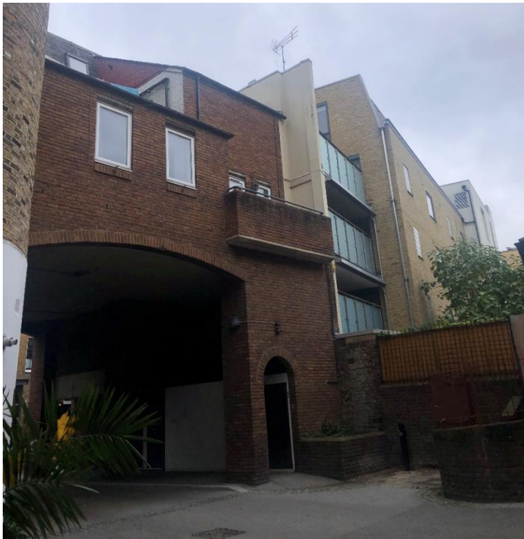
5. Rear of the application building showing undercroft area.
