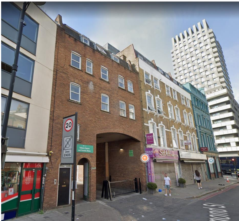
4. Front elevation of the application site.
