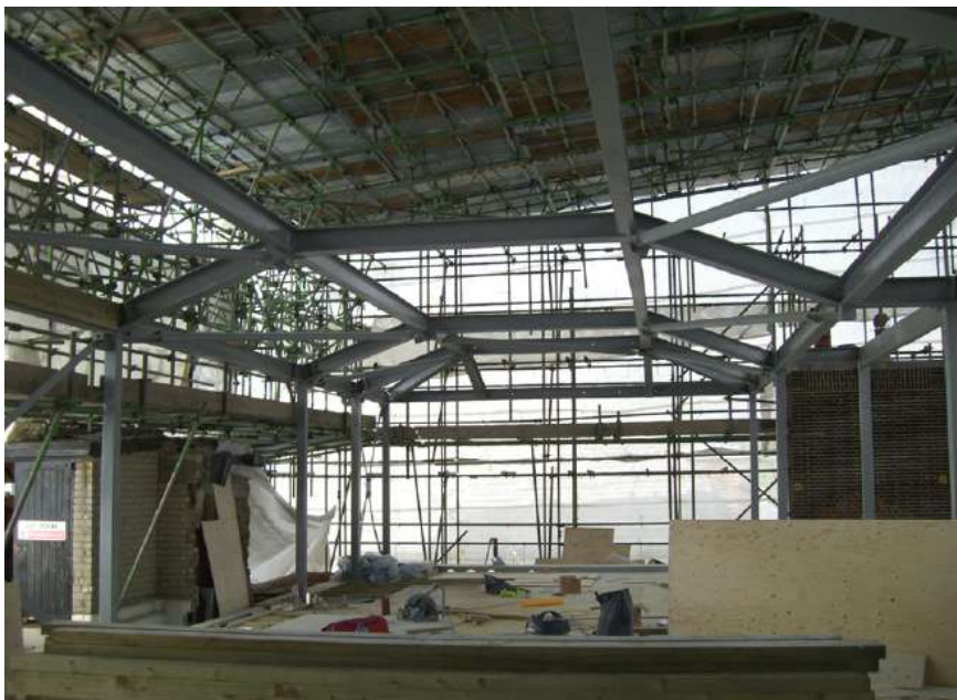
Photo 5: Primary structure erected above transfer deck on MBP's Lowndes Square penthouse.
