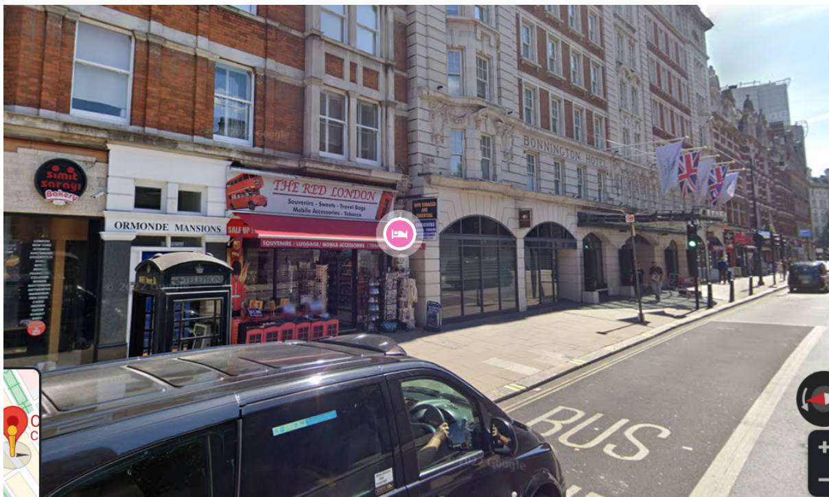
Site situated in a busy commercial area with numerous ground floor commercial uses
