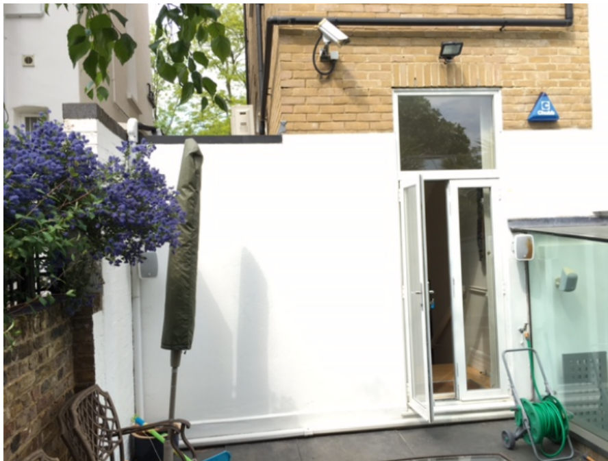
4. Photo extract from Members Briefing Pack at the application site under app ref 2017/1916/P.
