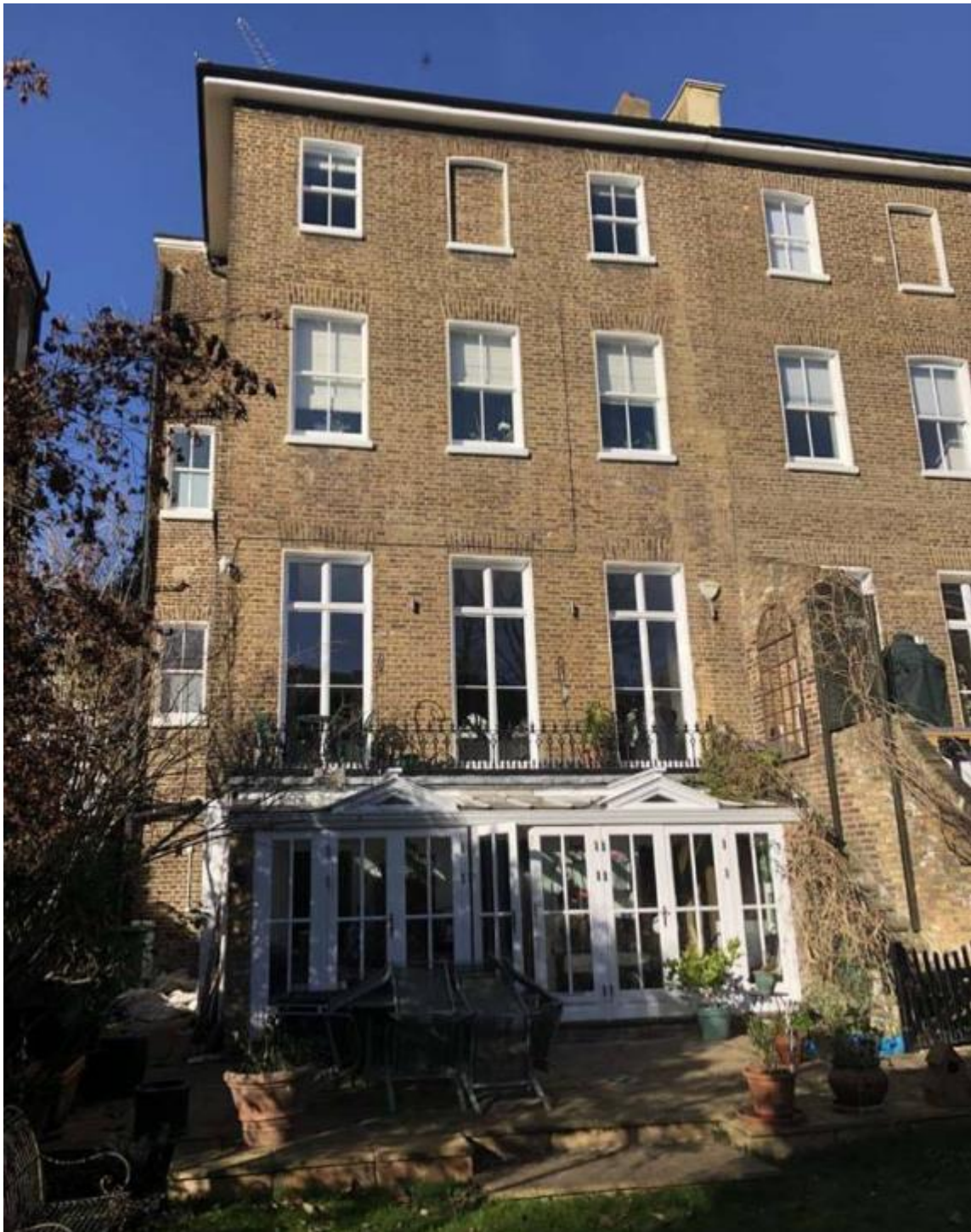
Photo 3: Photograph of existing rear façade of 31 Buckland Crescent (above)
