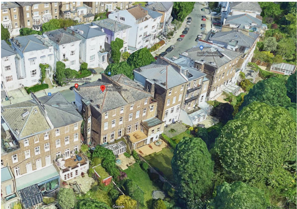
Photo 2: Close-up aerial view of rear of 31 Buckland Crescent (above)
