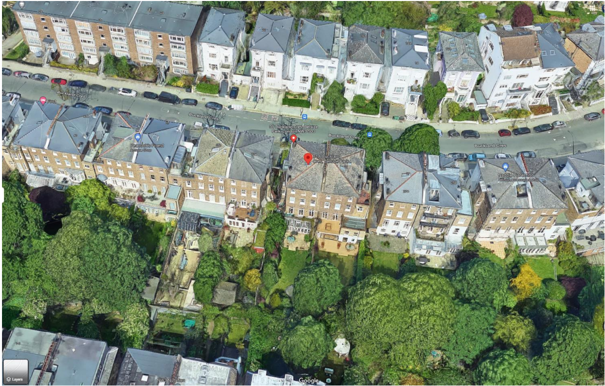
Photo 1: Aerial view of rear of 31 Buckland Crescent (above)
