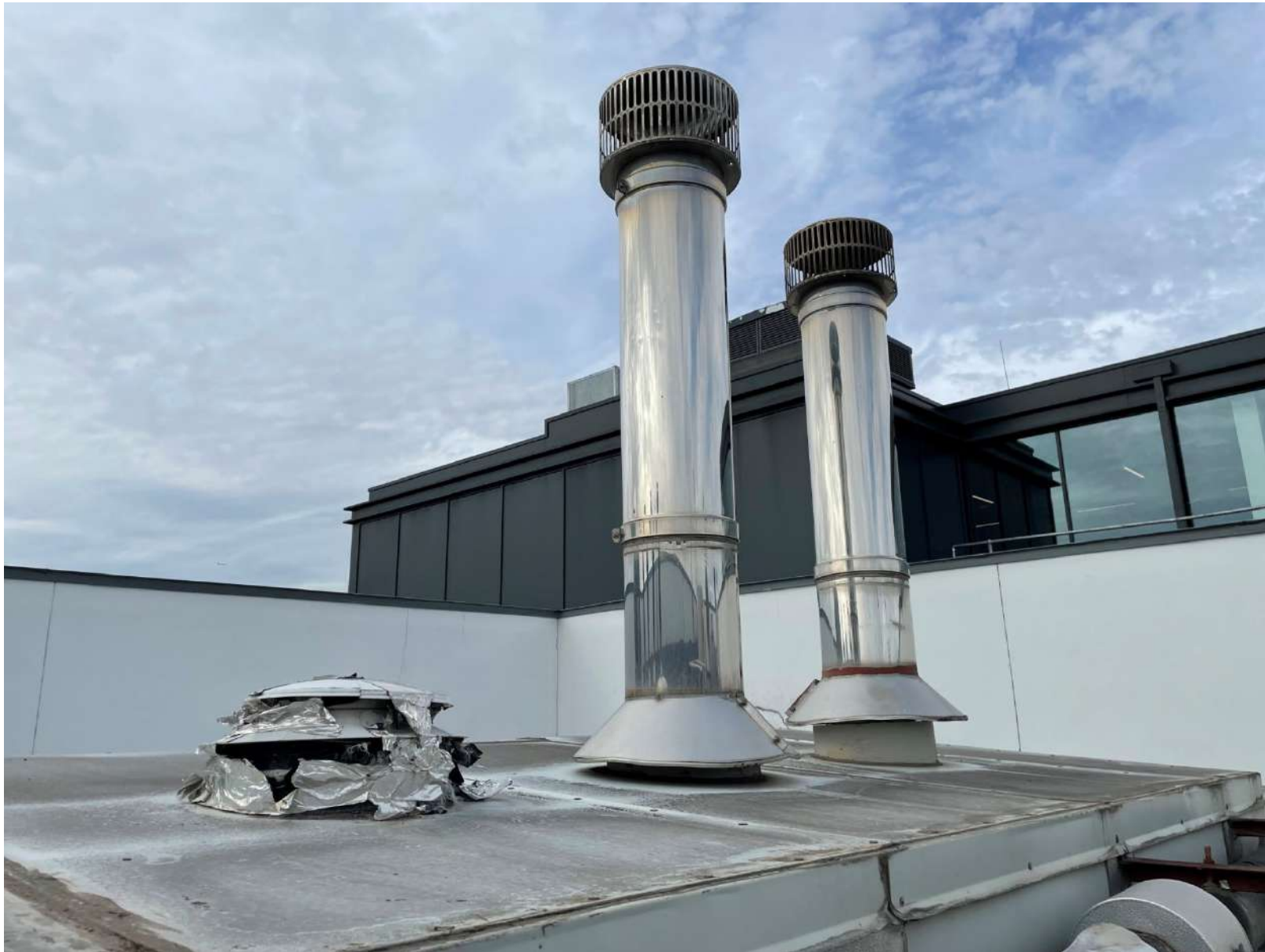
Photo J - Existing boiler flue terminals above the boiler house inside the fifth floor plant compound
