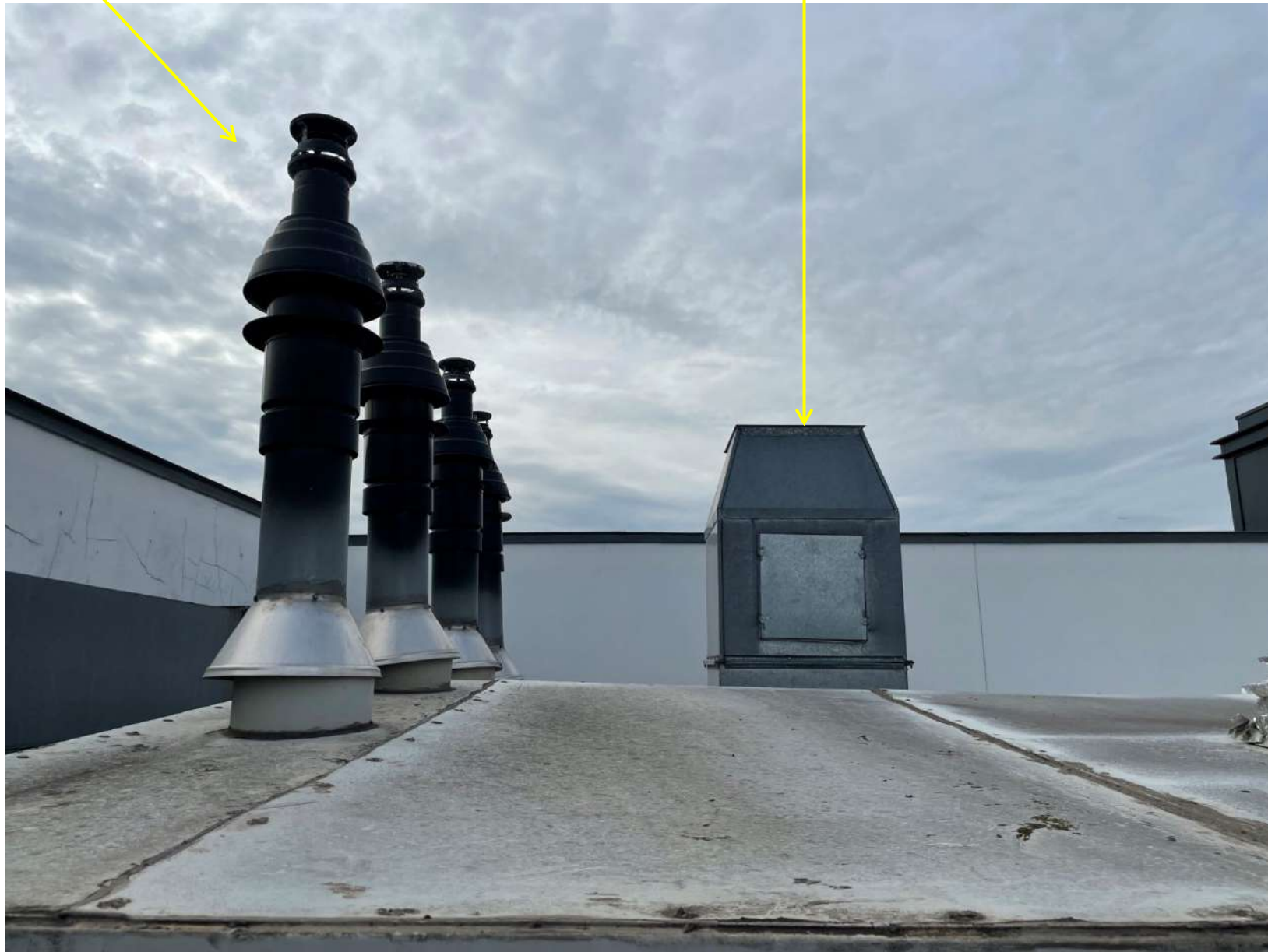
Photo K - Existing terminals above the boiler house inside the fifth floor plant compound
