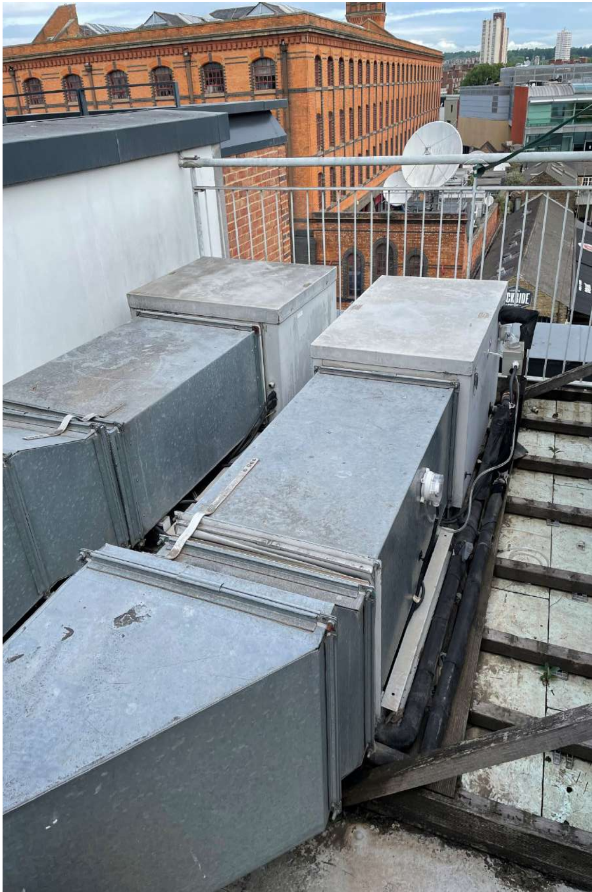
Photo G - Existing Extract ventilation units at the rear on the West side of the Hotel roof
