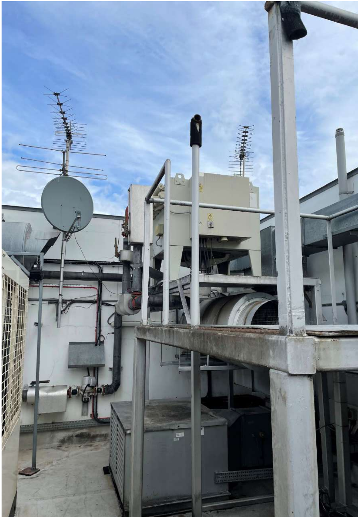
Photo I - Air cooled condenser at high level inside the existing fifth floor plant compound
