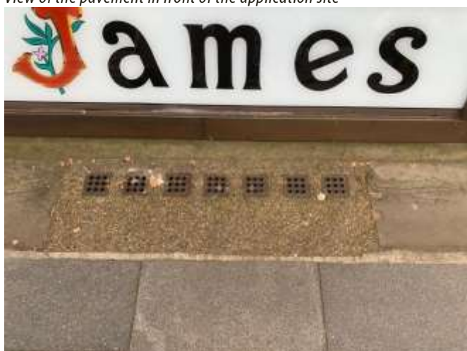
Ventilation cast iron blocks set in the concrete
