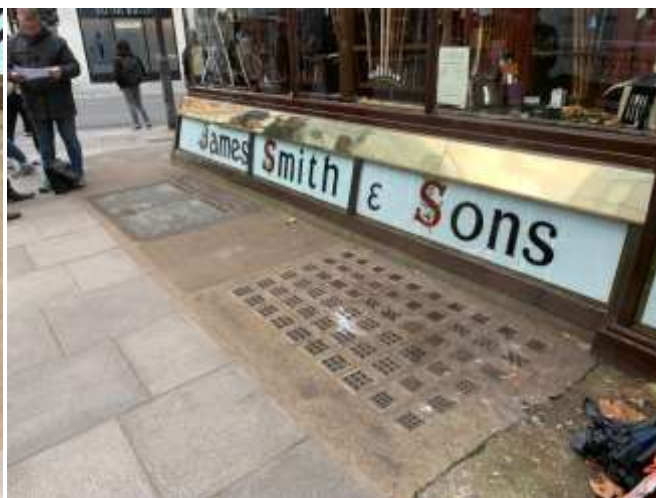
View of the pavement lights
