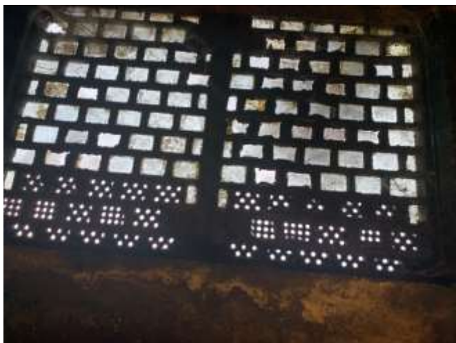
View of pavement lights from below
