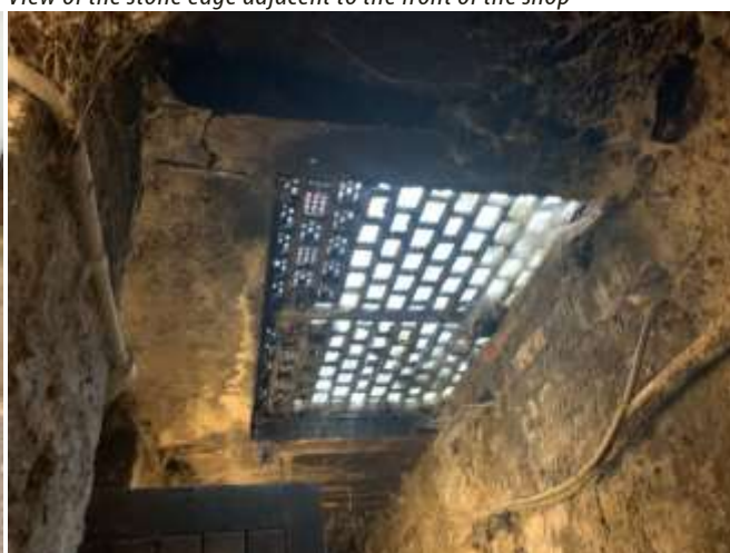
View of the pavement lights from below
