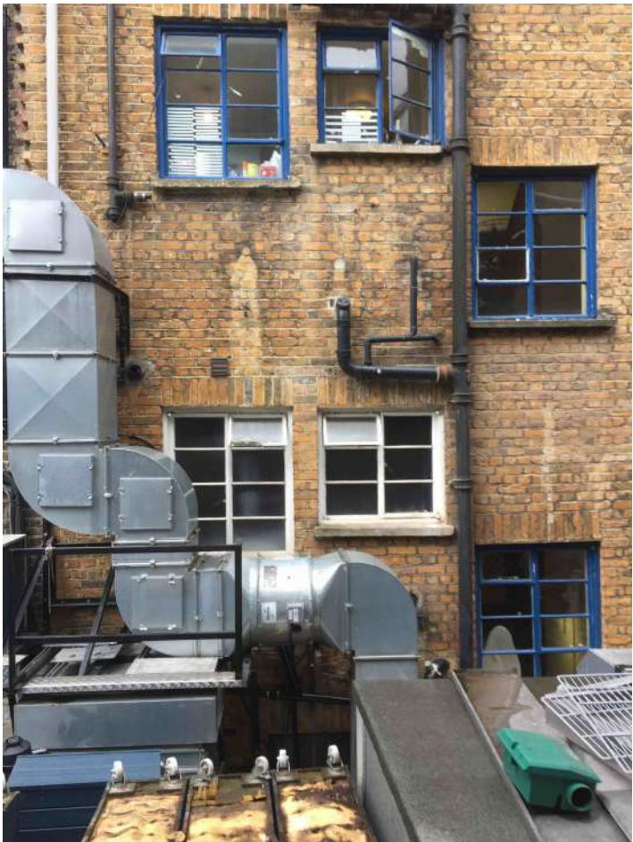
Image 6) Detail of lower portion of rear elevation of No. 82. Ventilation ductwork serves the kitchens to the Punjab'
