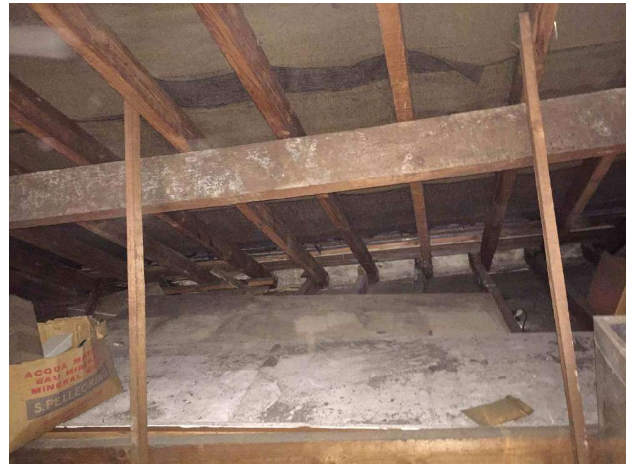
Image 15) View within roof void of No. 82 showing rafters, purlins and support struts (not original).
