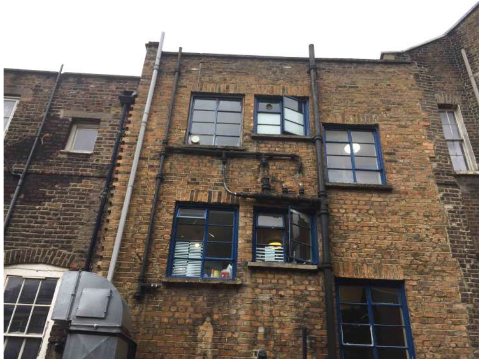
Image 3) Rear elevation view of 82 Neal Street upper portion with existing Crittall windows.
