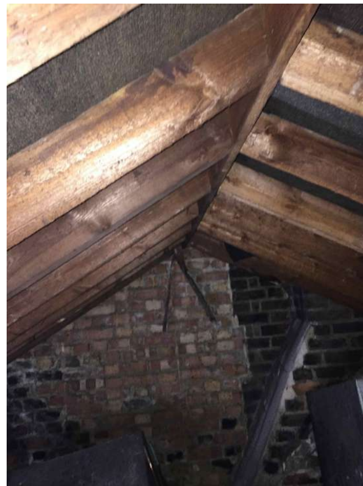
Image 14) View within roof void of No. 82 showing roof construction and party wall with not original roof structure and construction (unlike roof of No.80).
