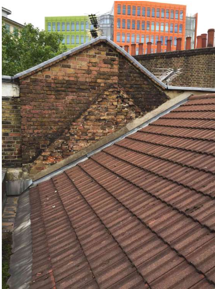
Image 8) View looking north from Roof of No. 82 to party wall between Nos. 80 and 190 Shaftsbury Avenue (Neal Street side). Note the concrete interlocking tiles, non original materials and that the roof form not being original. The roof was reconstructed following war damage.
