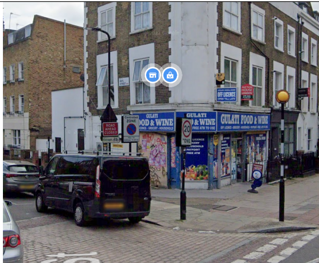
Figure 2 (above): Existing shopfront (including Rhyl Street elevation)
