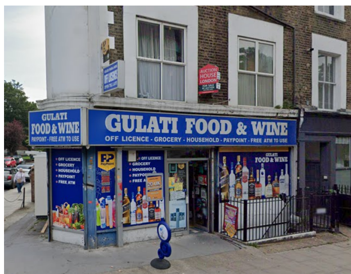
Figure 1 (above): Existing shopfront (Malden Road elevation)
