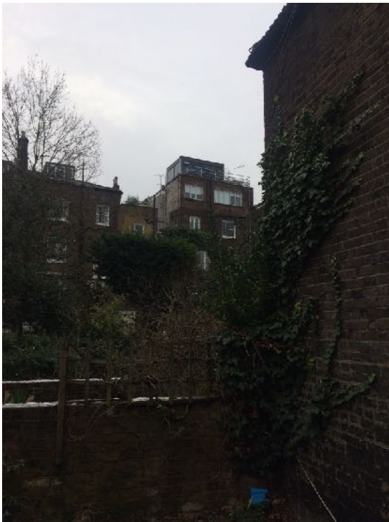
Image 6 Neighbouring Roof Structures
