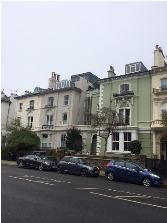
image 7 Neighbouring Roof Structures
