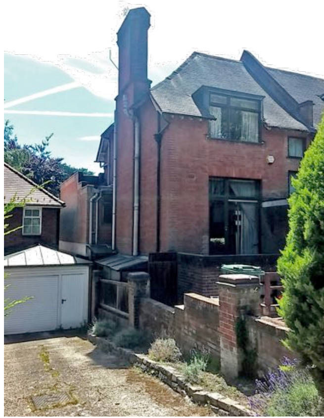
View from street at Nos.56 & 58a Redington Road
