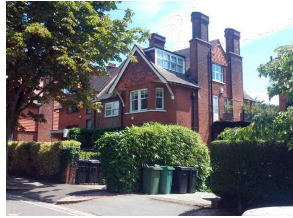
View from street at Nos.58, 58a & 58b Redington Road
