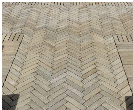
Vande Moortel Clay Pavers Laid on edge in a 45° Herringbone Pattern with an edging course in Soldier Bond.
