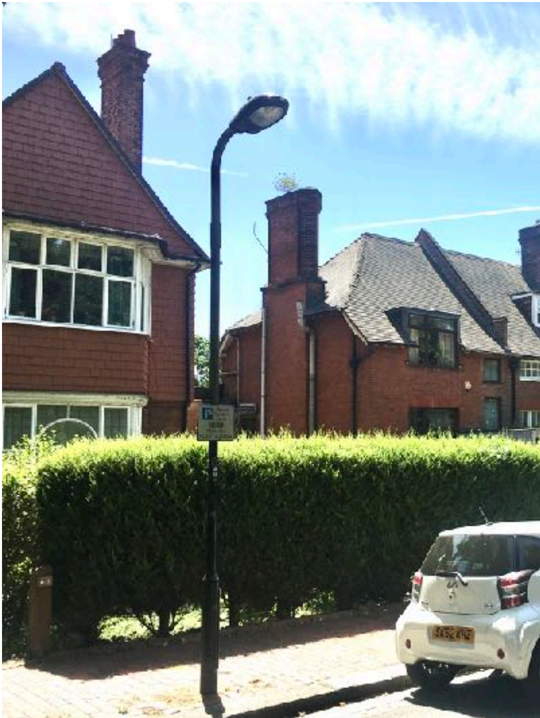
The original chimney stack, Photo 2 of 2:
