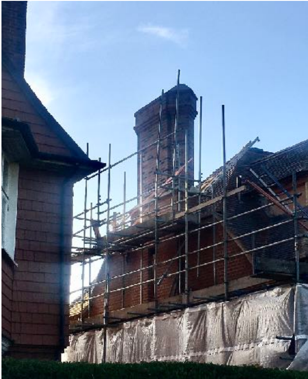
The rebuilt chimney stack, Photo 1 of 1:
