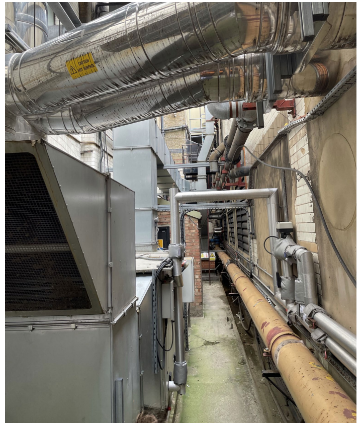
2. Photo of existing external passage on south east elevation that accesses location of window
