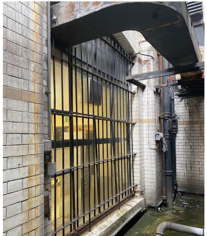
Photo of the window to be replaced
