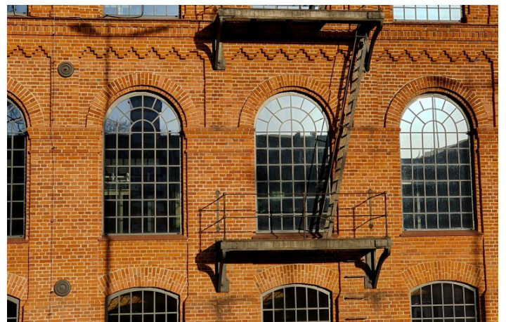
Photo of W20 steel frame window in brick wall
