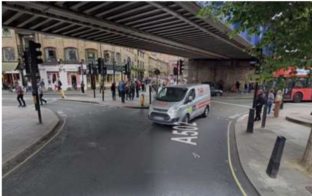
Figure 6 – View showing one way system away from the northeast on Castlehaven Road
