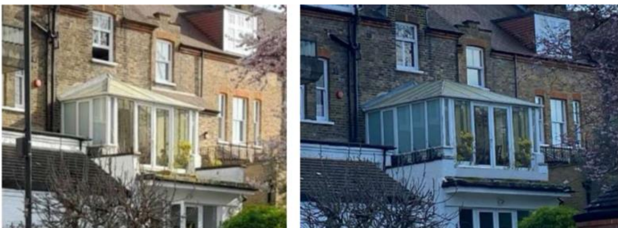
Figure 1 (above): Extract images taken from page 13 of the appellants statement of case
