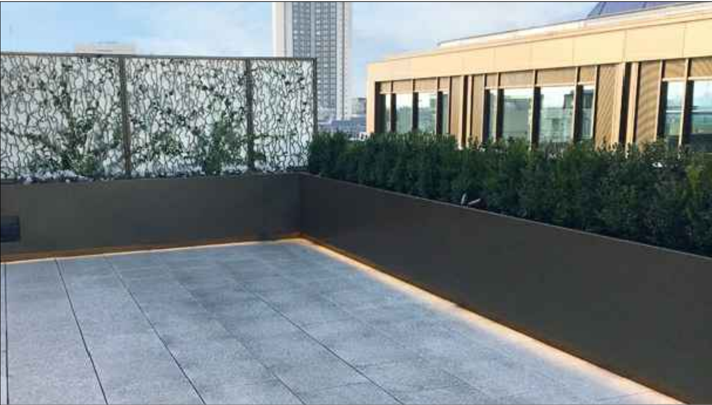
F22 Bespoke Mild Steel Planter MANUFACTURER: Kinley RANGE: Perimeta Planterline Bespoke WEBSITE: www.kinley.co.uk MATERIAL: 3mm folded mild steel panel system powder coated to RAL 7016 FIXING: Fixed to roof tray
