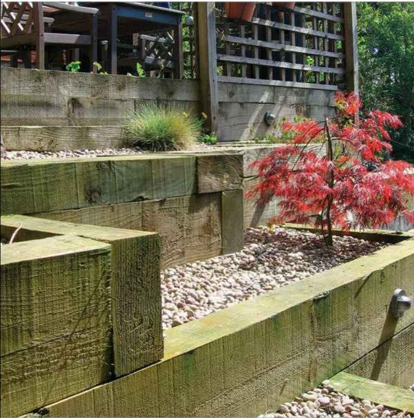
F14 Bespoke Timber Raised Sleeper Bed MANUFACTURER: UK Sleepers PRODUCT: New European Softwood (Larch/ Douglas Fir) Railway Sleeper FINISH: Smooth finish, Incised Green Pressure Treated Sleeper. DIMENSIONS: 2400mm x 200mm x 100mm FIXING: Fixed to roof tray
