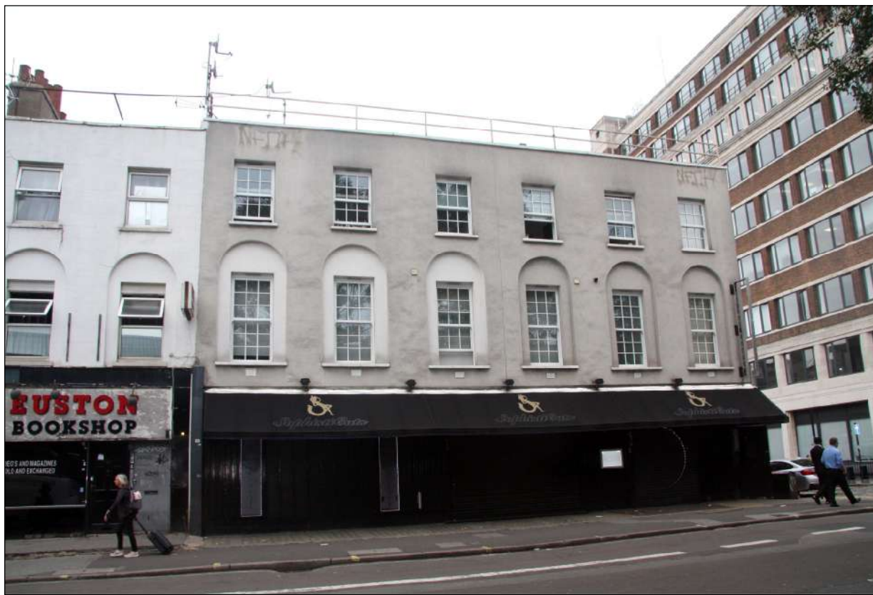
Plate 5) Principal facade as seen from Eversholt Street
