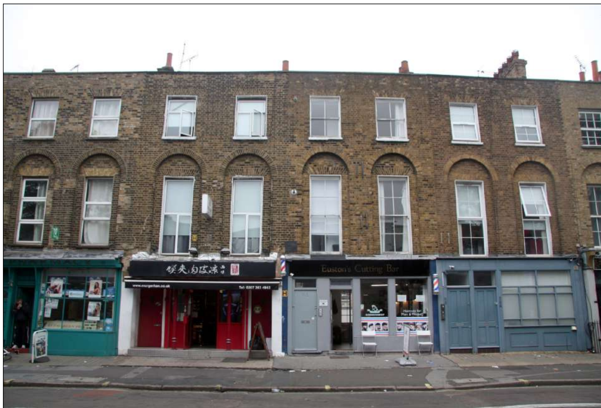
Plate 21) View of 64-58 Eversholt Street
