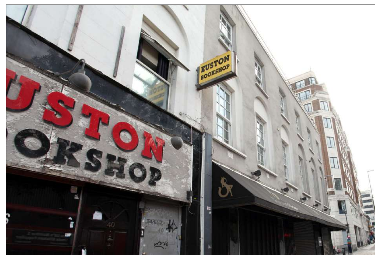
Plate 24) Site and Euston House as seen from Eversholt Street
