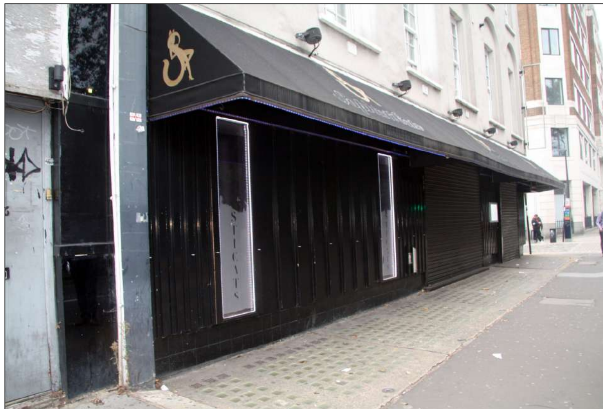
Plate 7) Shop front with modern notice boards, entrance and openings
