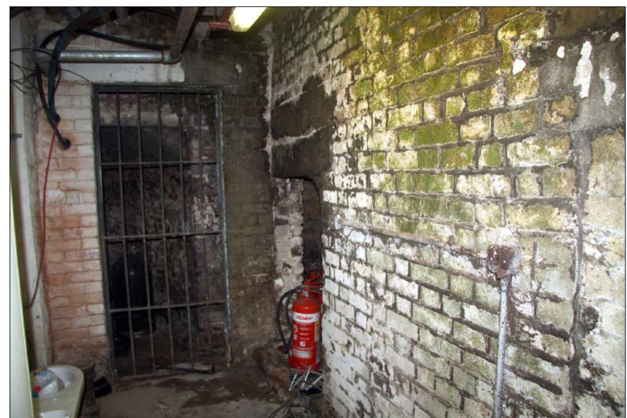
Plate 16) View of vaulted storage area and corridor of basement, beneath pavement
