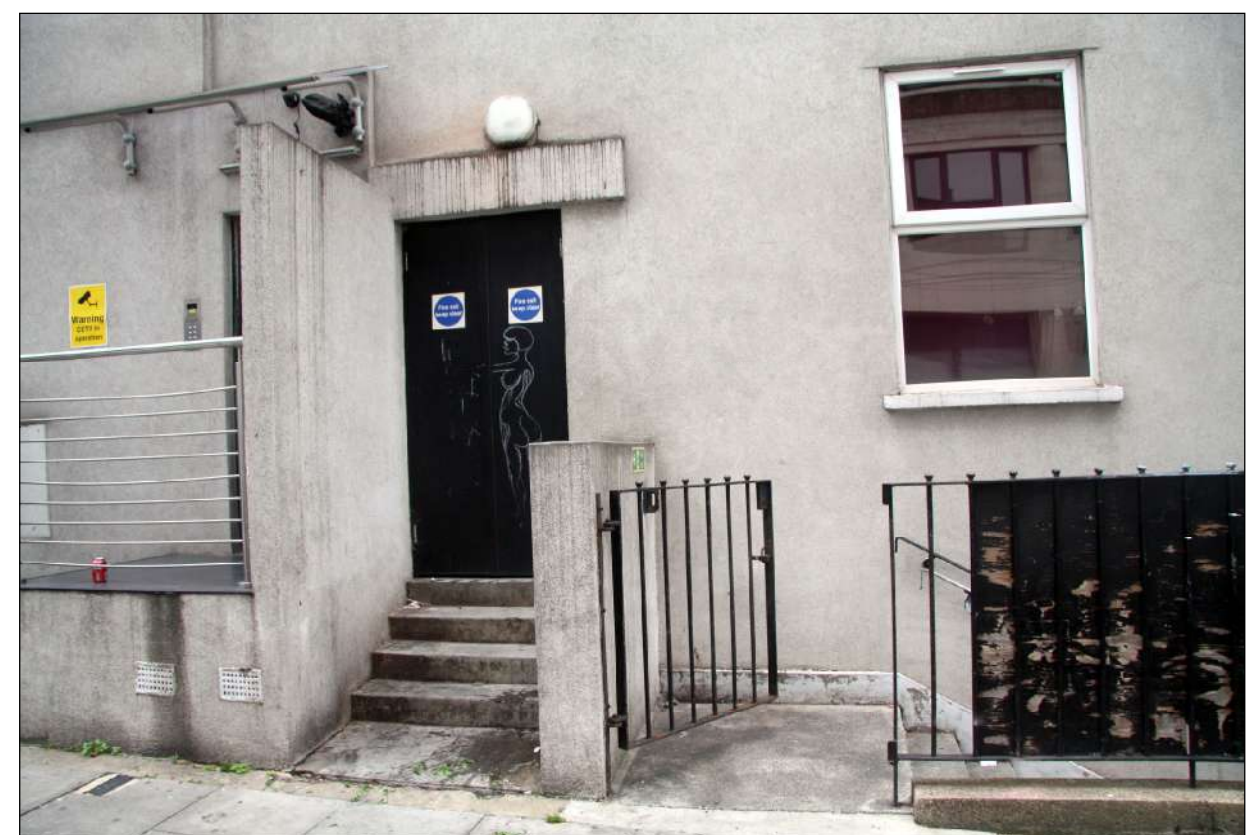
Plate 12) Fire exit from Doric Way
