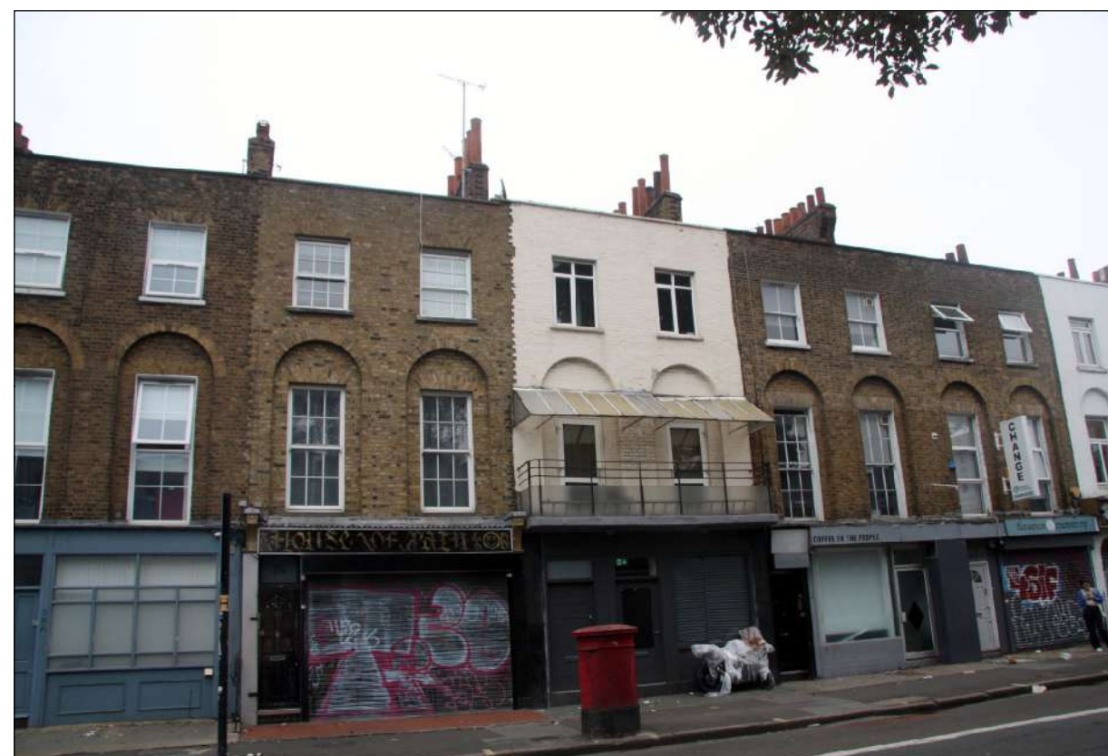
Plate 22) View of 56-50 Eversholt Street
