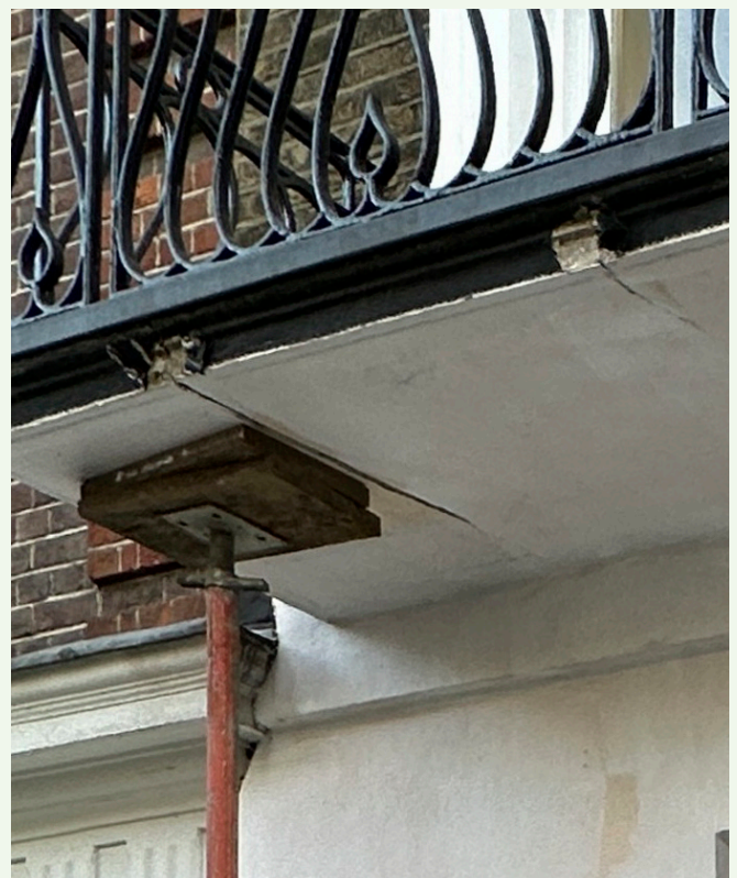
Fig B - Existing cracks to underside of balcony
